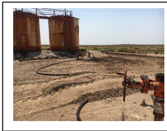
Equipment Area after scrapping
