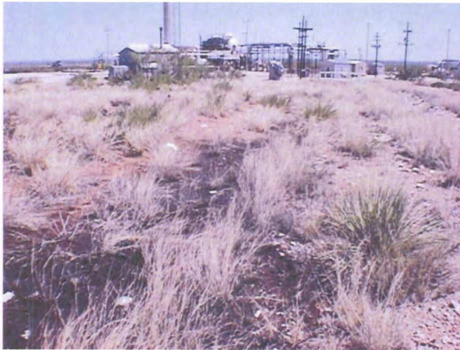
Chevron #214 Leak Site – Facing Northeast, July 1998
