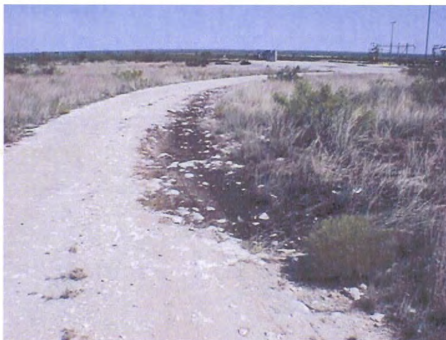
Chevron #214 Leak Site – Facing North, July 1998
