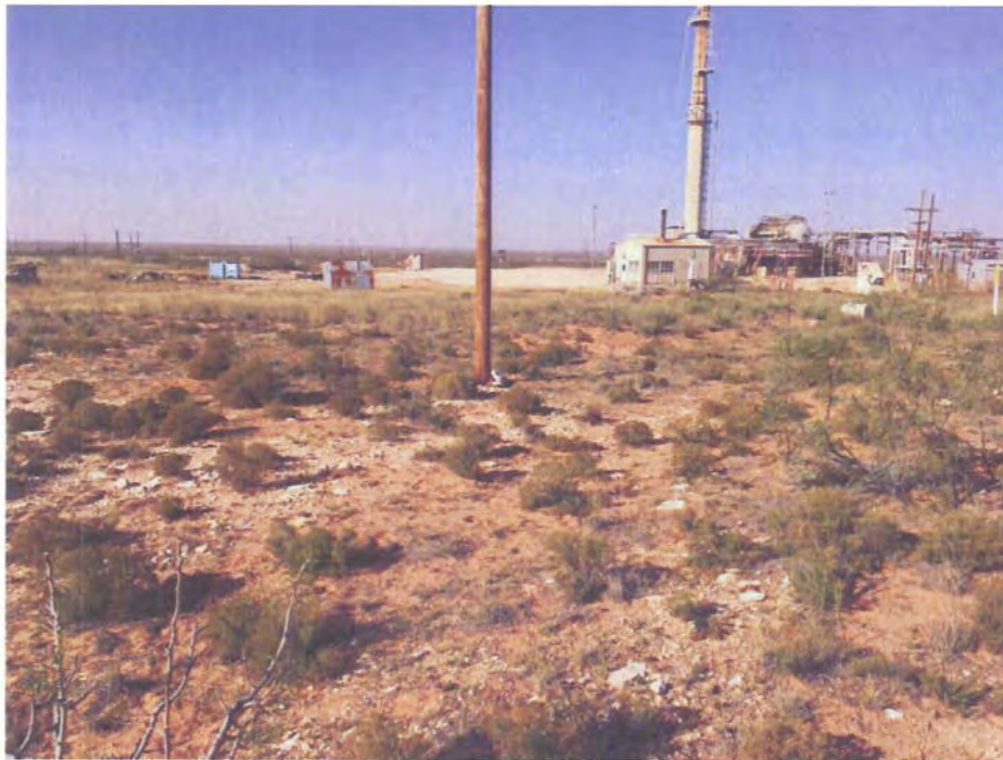
Chevron #214 Leak Site – Facing North, November 2017
