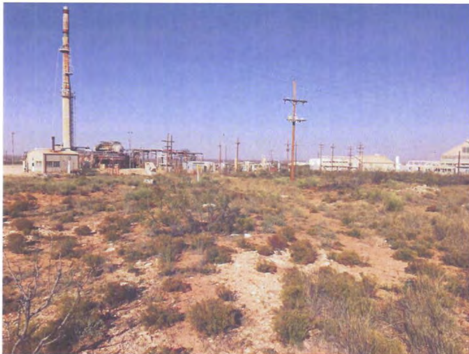
Chevron #214 Leak Site – Facing Northeast, November 2017
