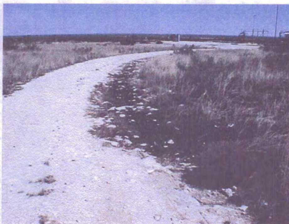
Chevron #214 Leak Site - Facing Southwest
