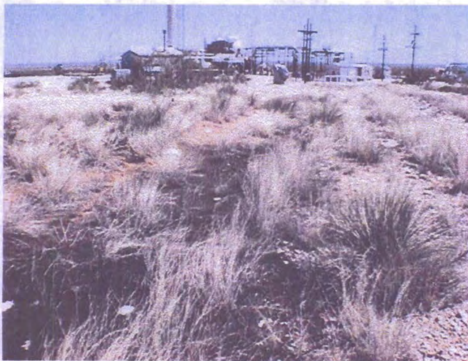
Chevron #214 Leak Site - Facing South
