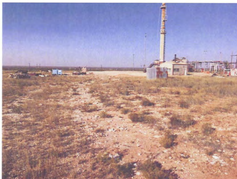
Chevron #214 Leak Site – Facing North, November 2017
