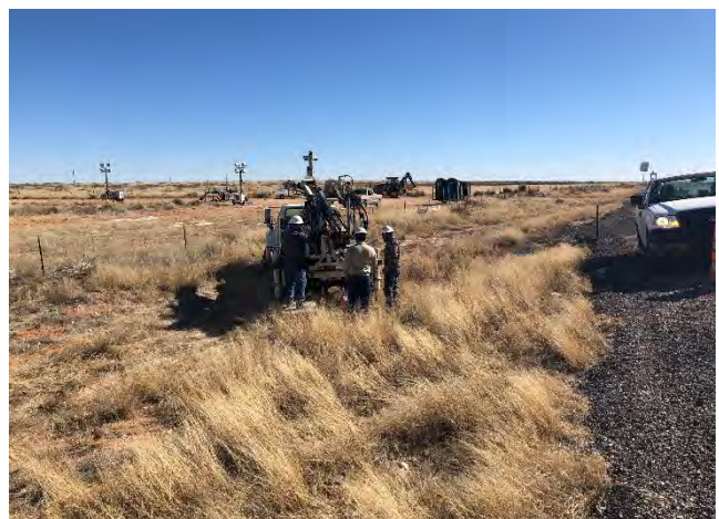
6. Typical view of boring installed via flight augers.
