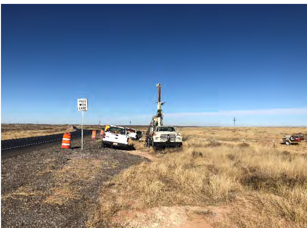
5. Typical view of a soil boring installed via flight augers within the ROW.
