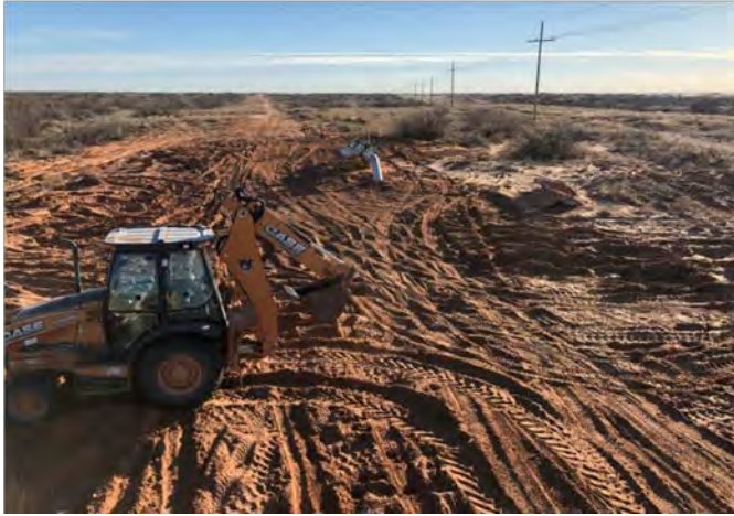
Photo 1: View of the excavation area.
