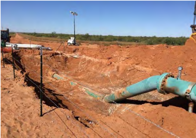
Photo 3: View of the excavation area, present prior to the spill.
