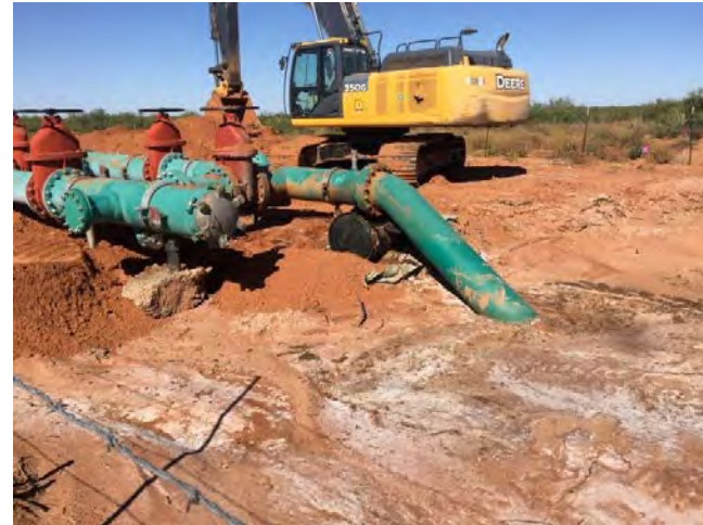
Photo 4: View of the excavation area, present prior to the spill. .
