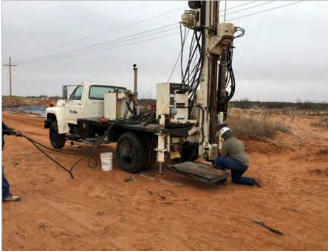
Photo 5: View of typical boring installed via geoprobe.
