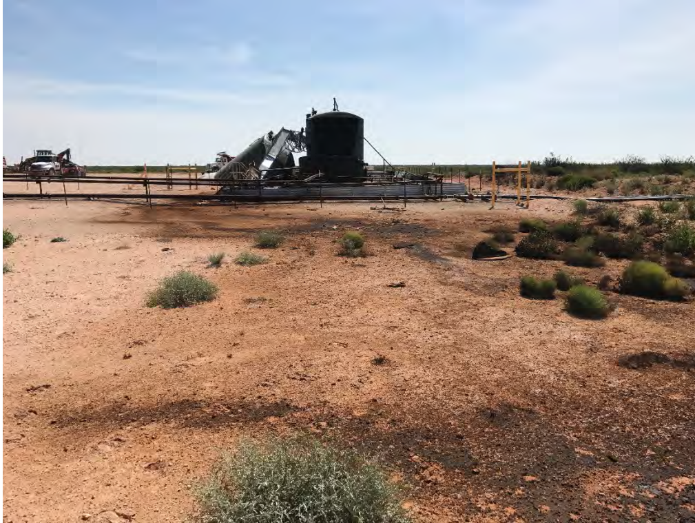
Madera 35 Federal #1H CTB – August 2017 Release (Looking East)
