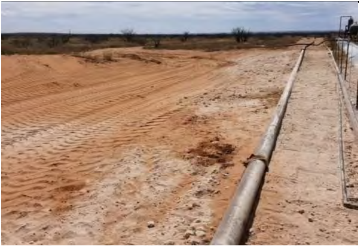
Figure 9 - View of the affected area after remediation activities, facing South.
