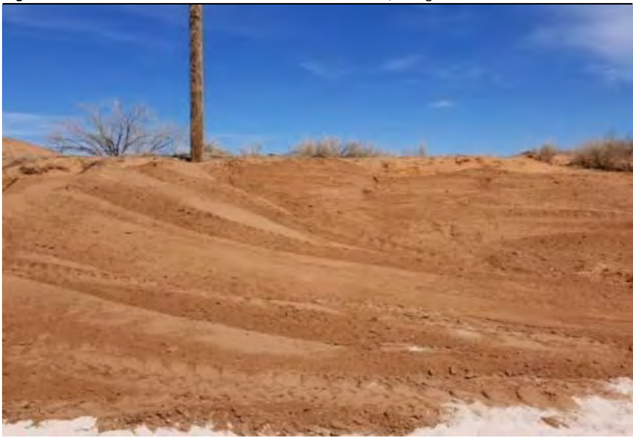
Figure 10 - View of the affected area after remediation activities, facing Northeast.
