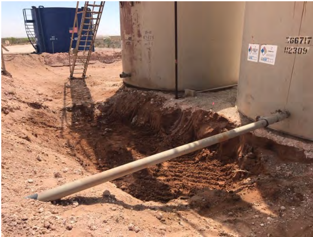
Excavation (Looking East-Southeast)
