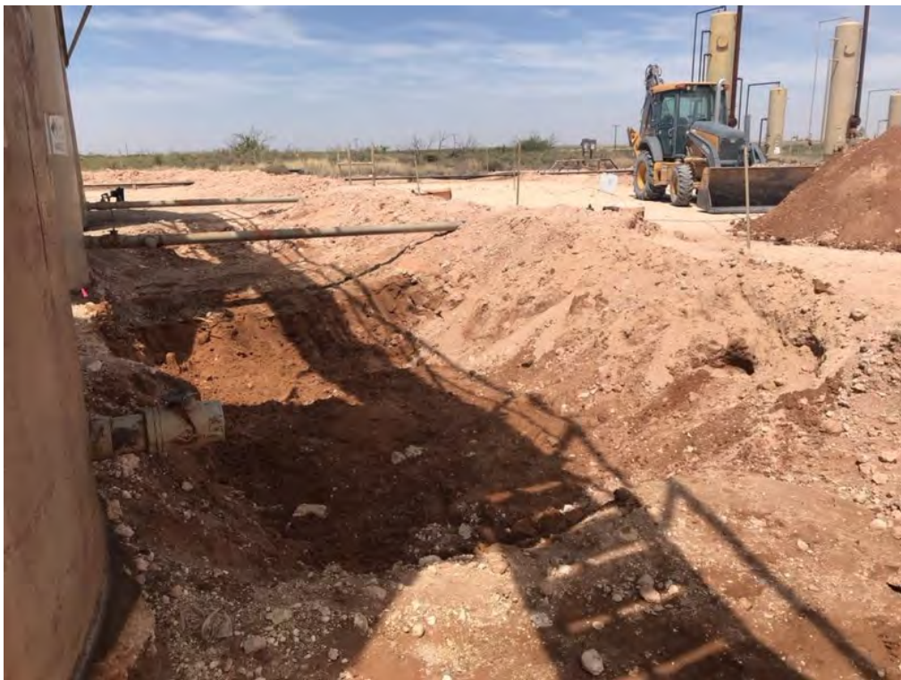
Excavation (Looking West-Northwest)
