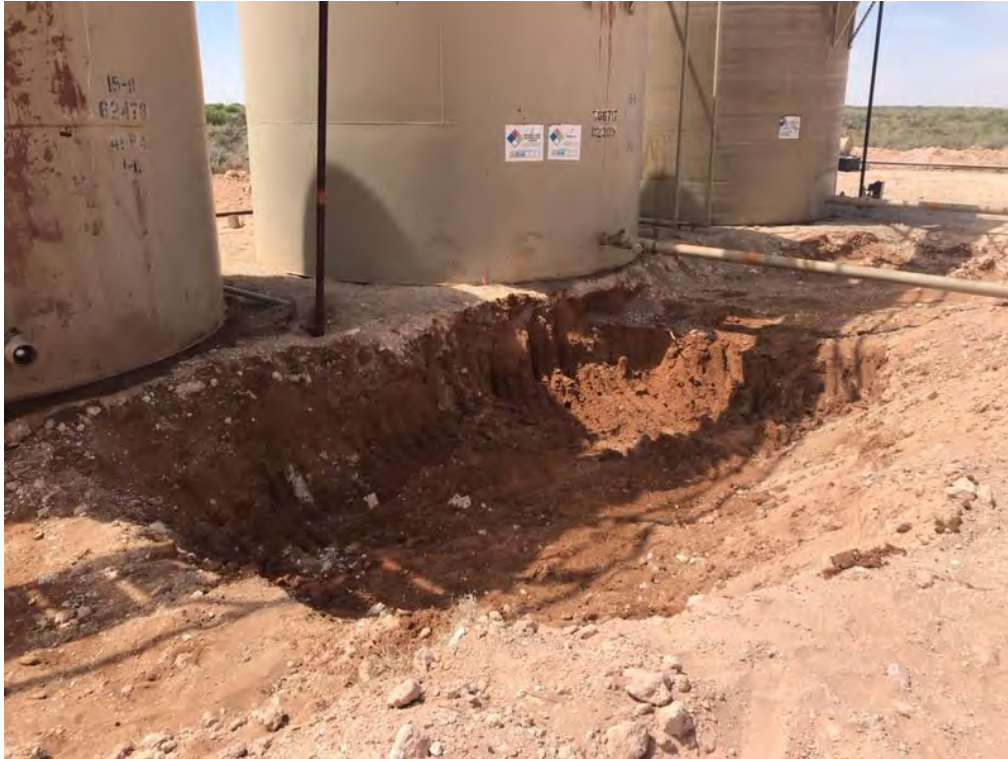
Excavation (Looking Southwest)
