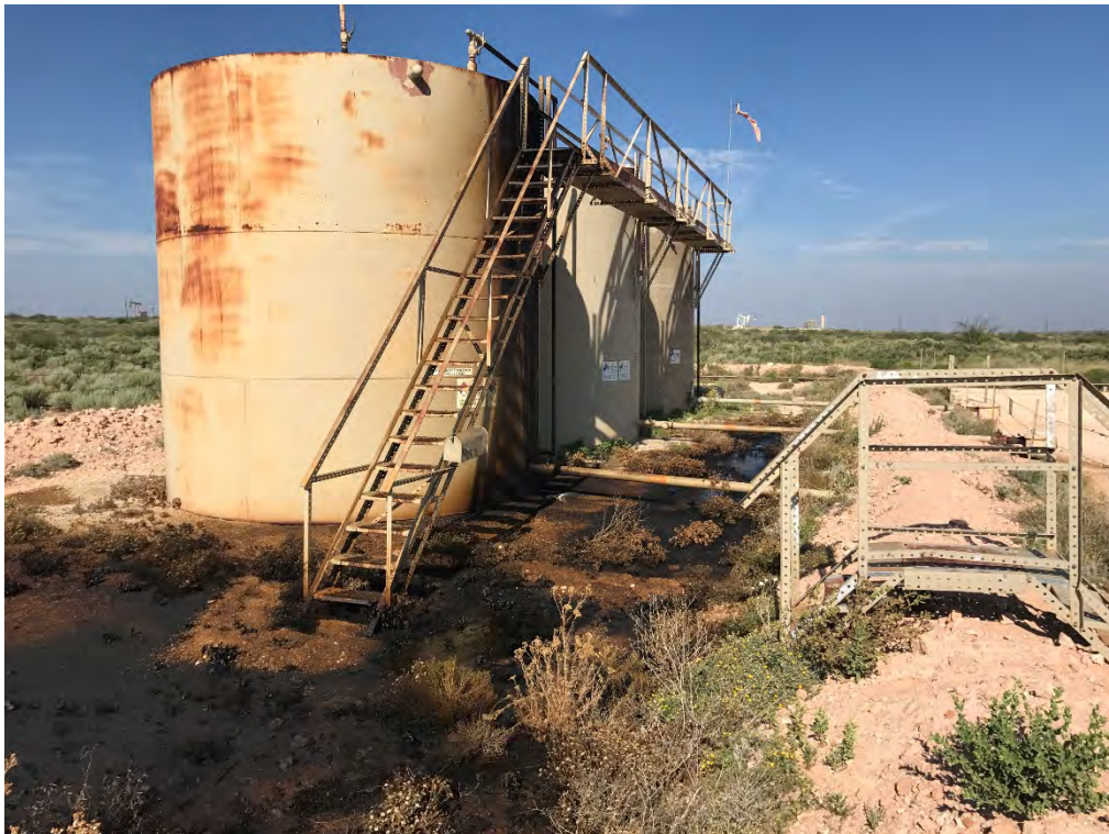
Release (Looking West-Southwest)
