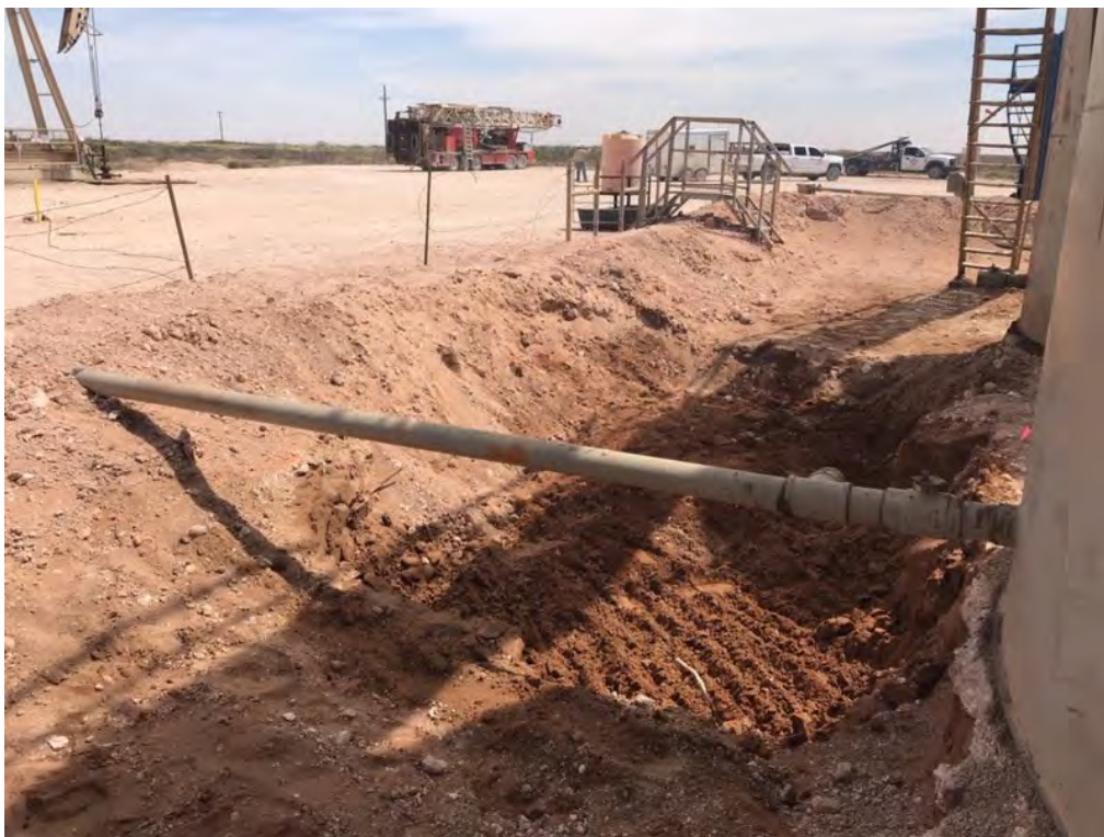
Excavation (Looking Northeast)
