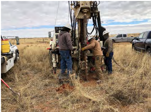
3. Typical view of borings installed via flight augers.
