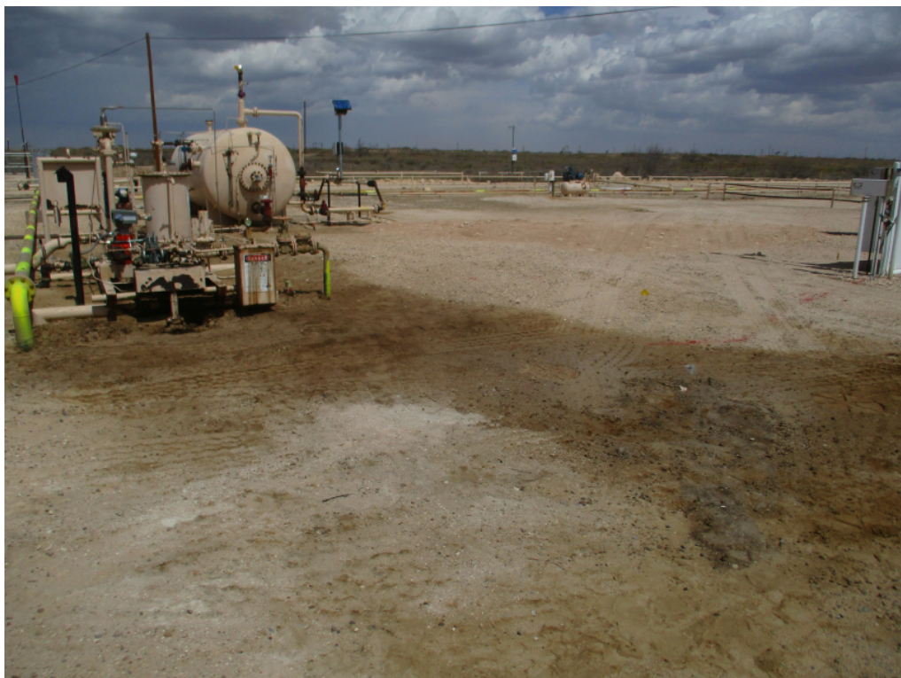
View Northeast– Area of BH-1
