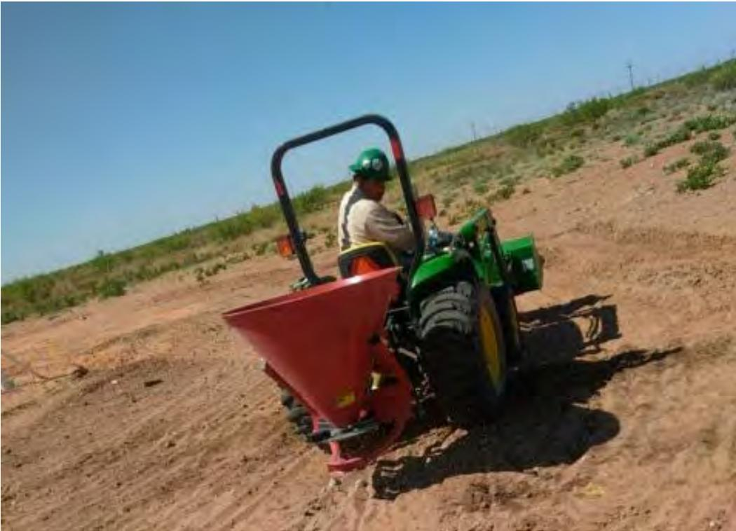
Photo 3 - Reseeding the backfilled excavation
