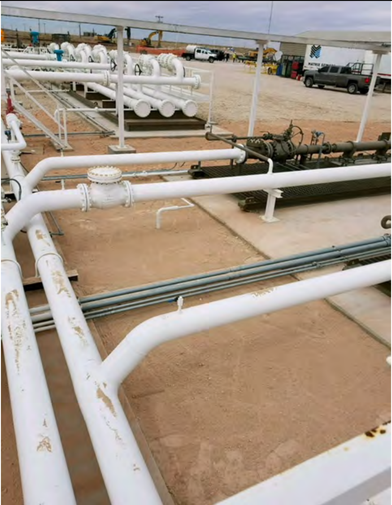
Photo 6: View of the affected area after remediation activities, facing northwest.
