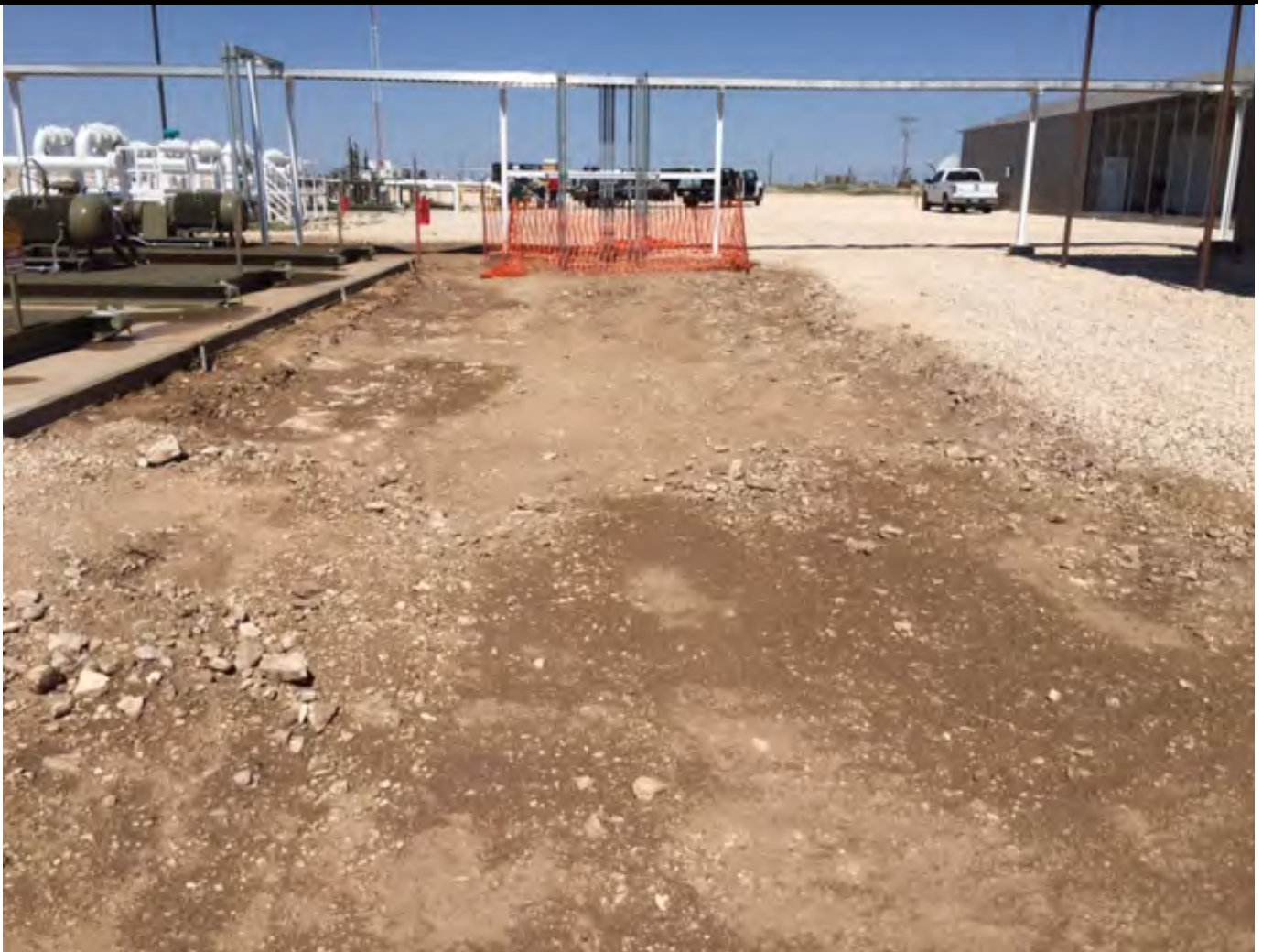
Photo 4: View of portion of excavated area, facing west.
