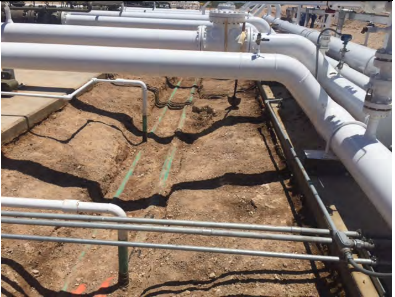
Photo 3: View of portion of excavated area, facing east.
