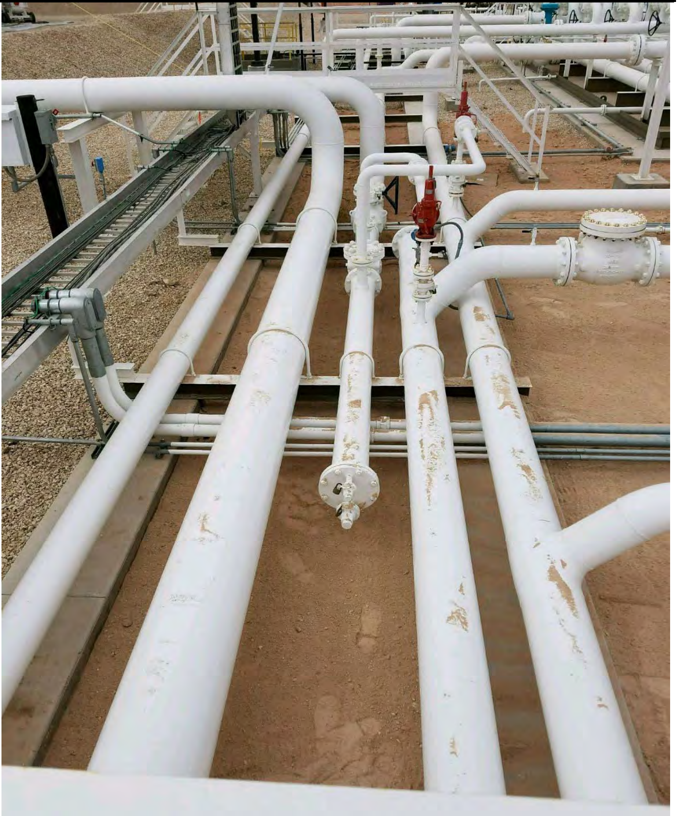
Photo 7: View of the affected area after remediation activities, facing west.
