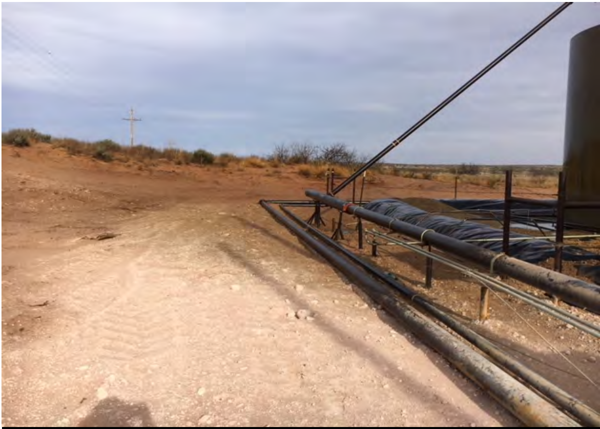
Figure 3 - View of overspray area, facing East.
