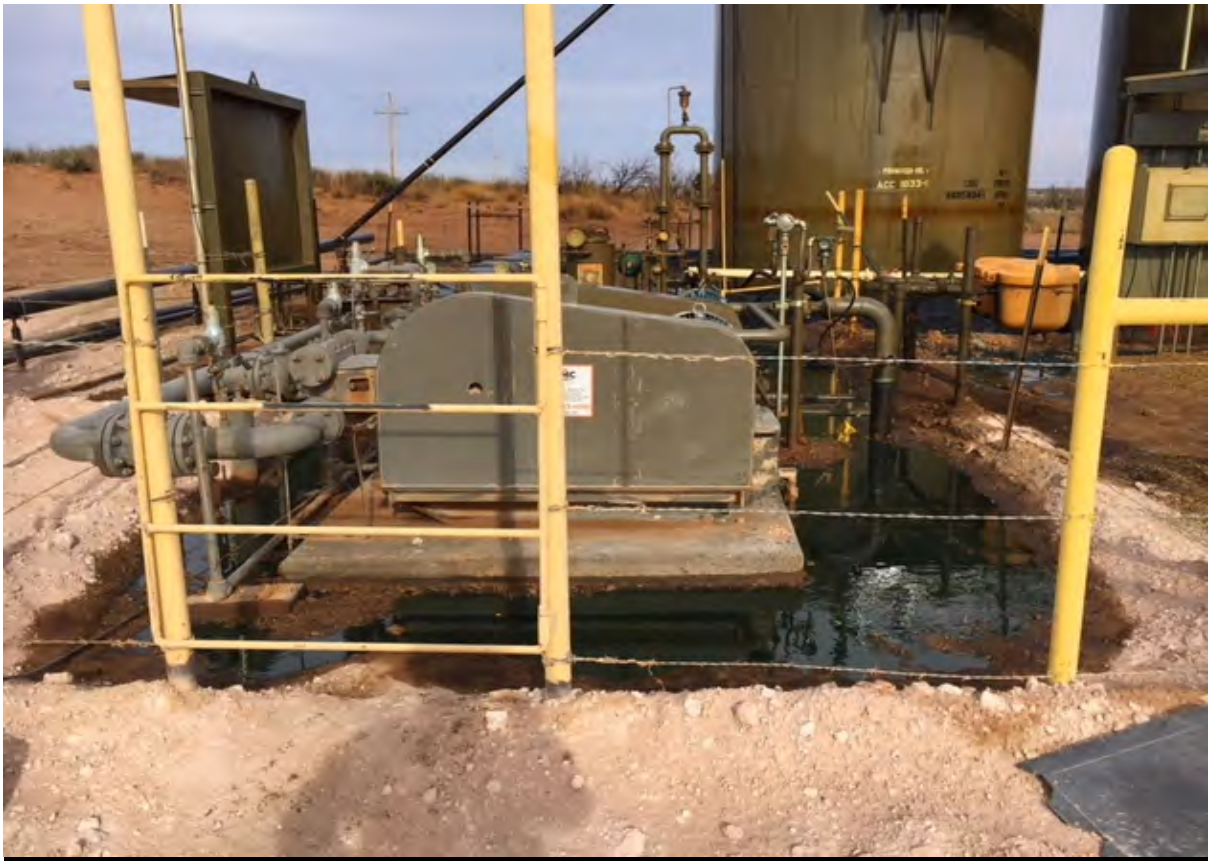
Figure 1 - View of the initial release, facing East.
