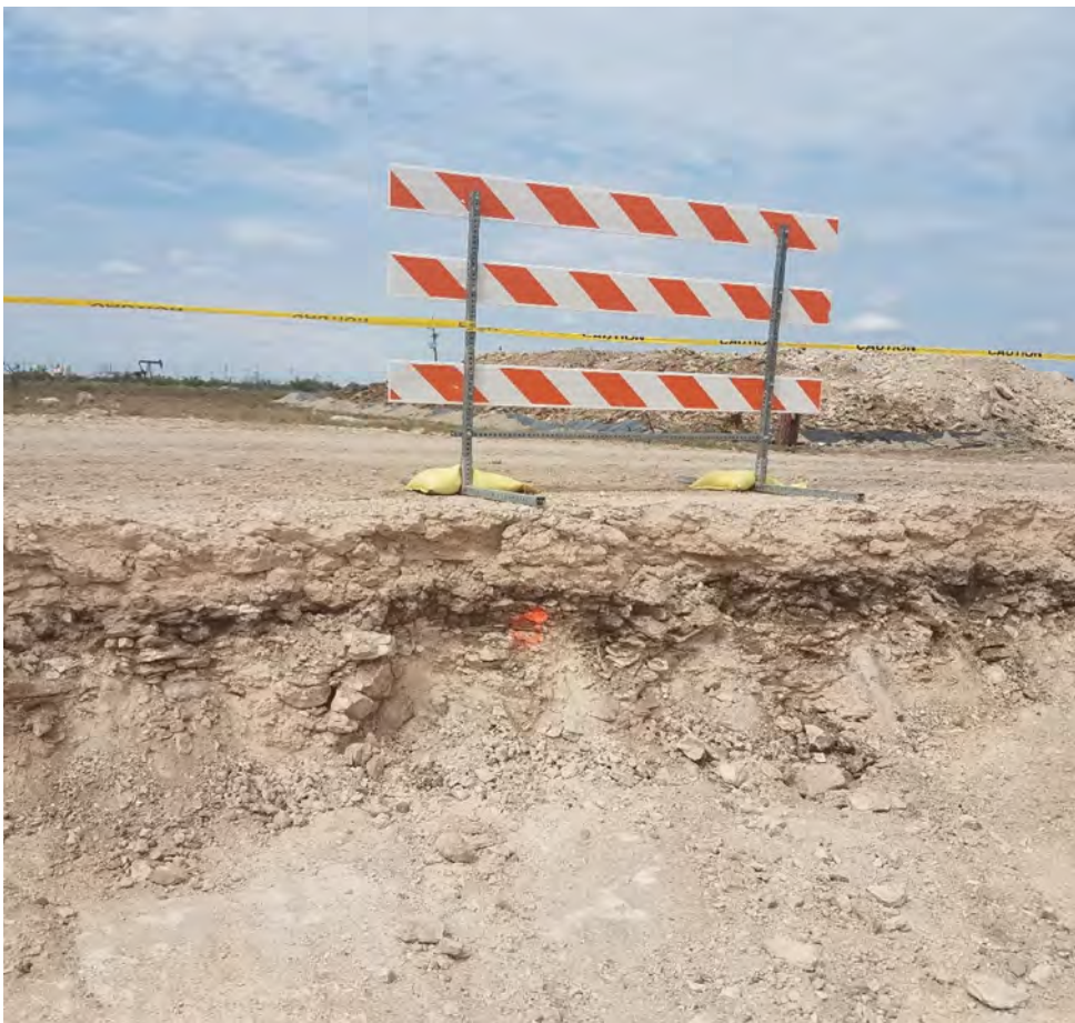
Photo 5: North end of release migration/excavation at north access road. Brown layer is soil. Looking north. August 10, 2018.
