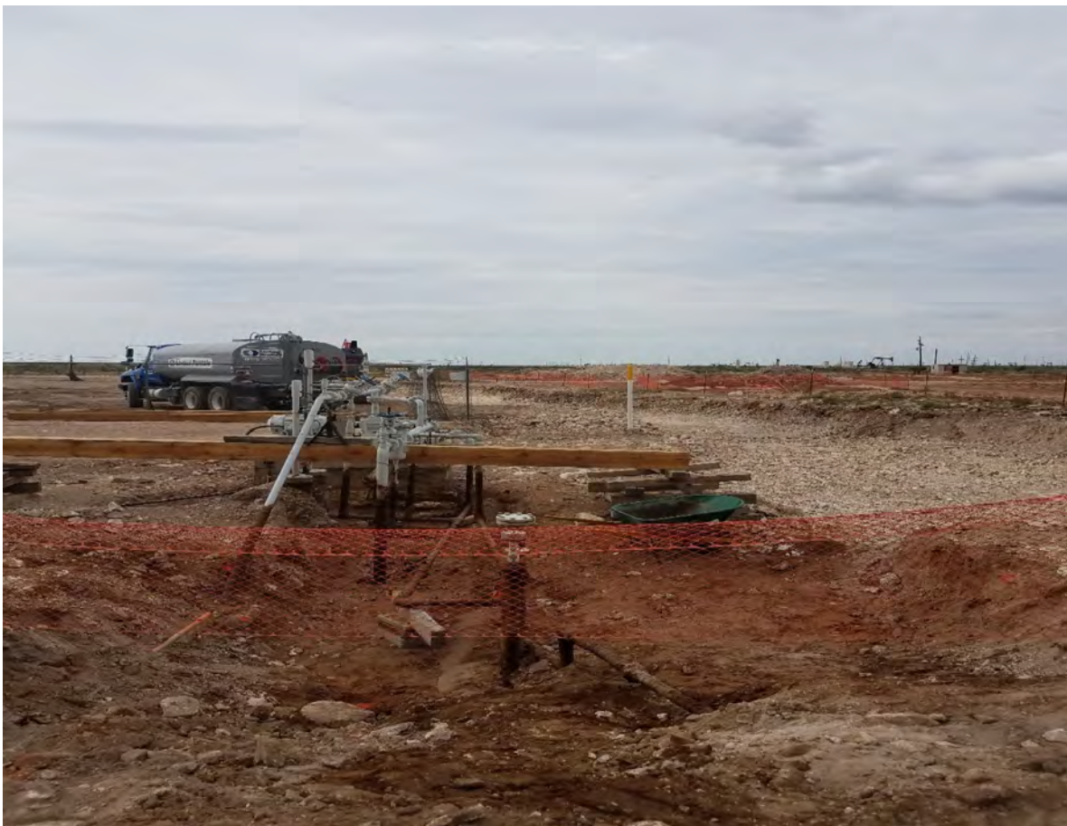
Photo 2: Pumping unit/sump excavation and lateral delineation to east and north. August 10, 2018.
