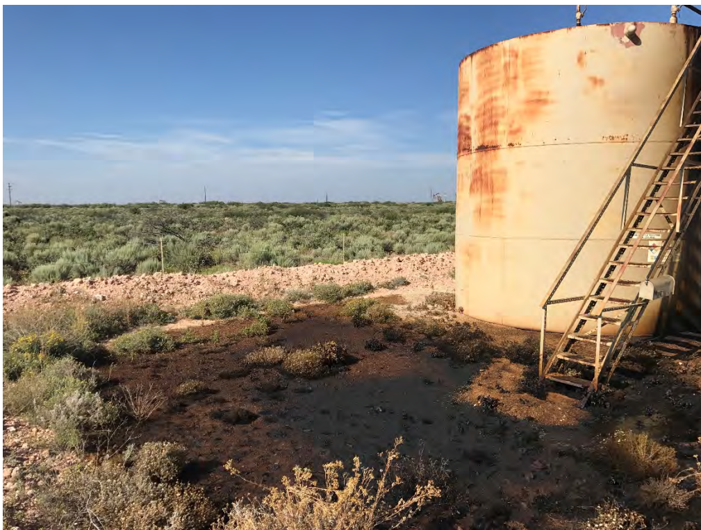
Release (Looking Southwest)
