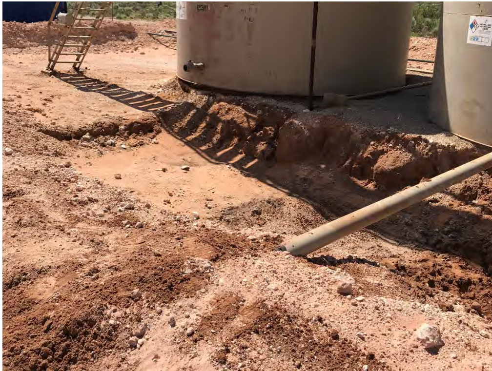
Excavation (Looking Southeast)
