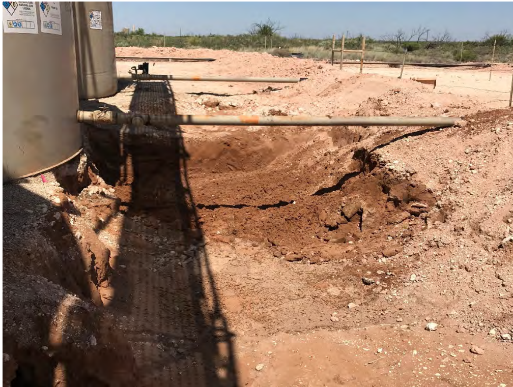
Excavation (Looking West-Northwest)
