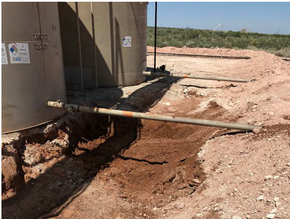
Excavation (Looking West-Southwest)
