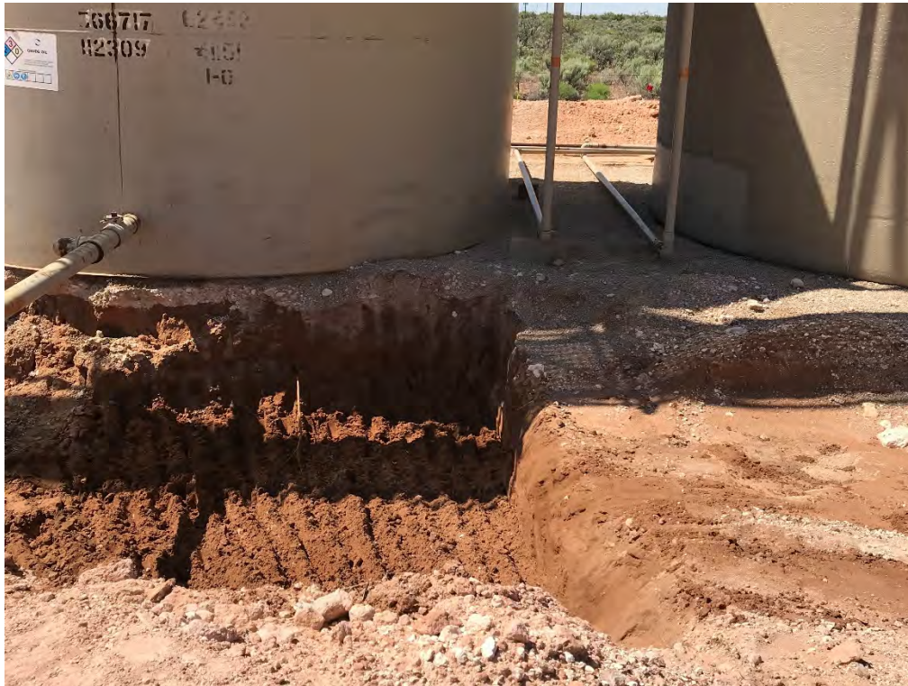
Excavation (Looking South)
