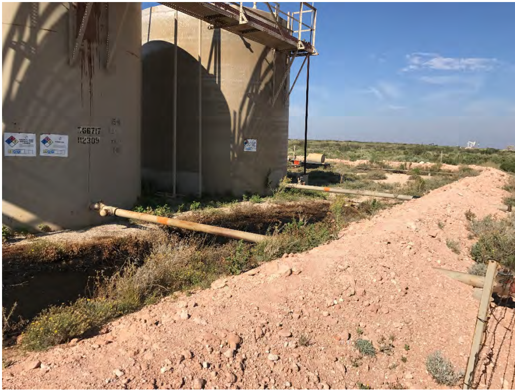
Release (Looking Southwest)
