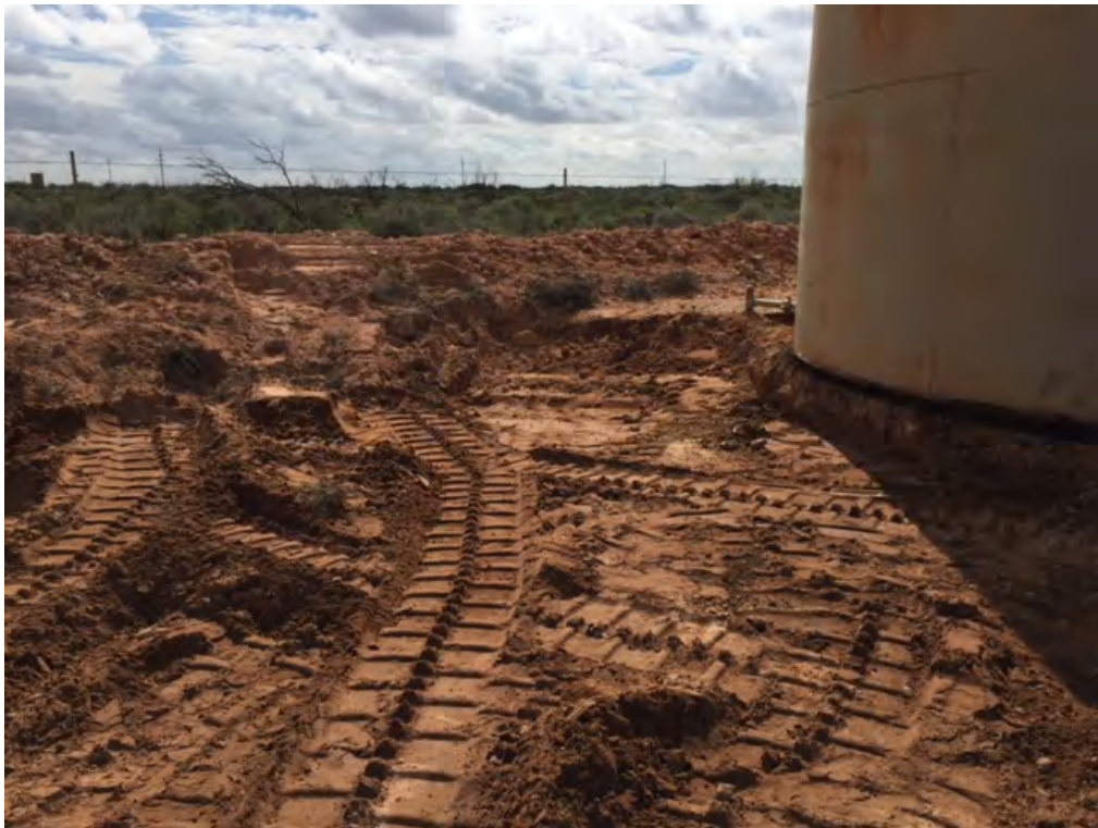
Excavation (Looking Southwest)
