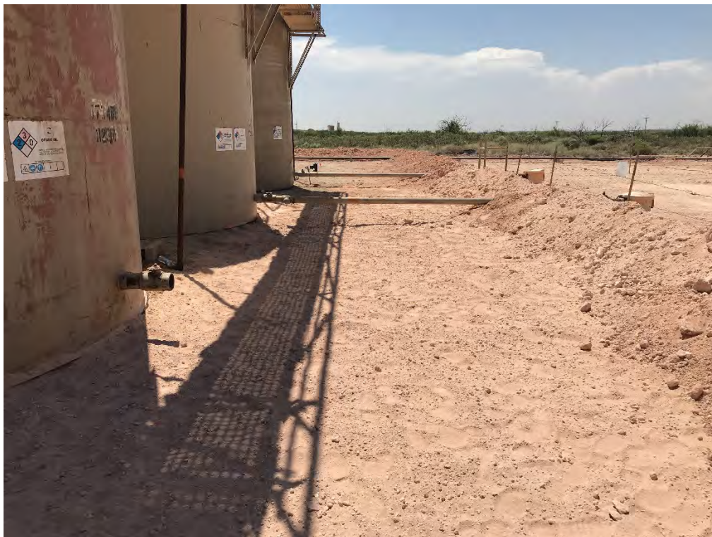
Backfilled Excavation (Looking West)
