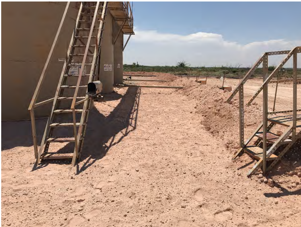
Backfilled Excavation (Looking West)
