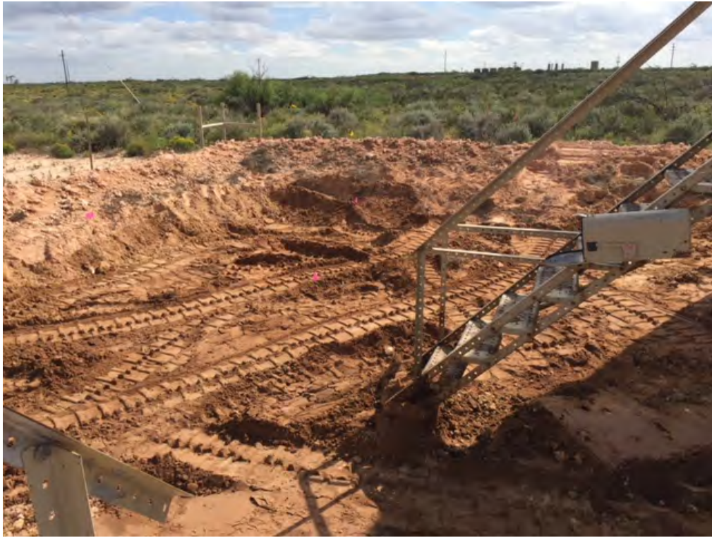
Excavation (Looking Southeast)
