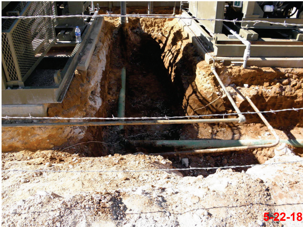
Photo 15 – View of hand digging activity around LACT Unit equipment facing north
