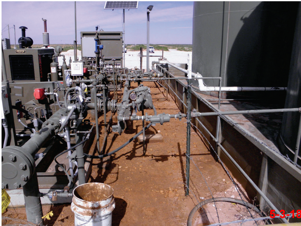
Photo 3 – View of impacted soil along northern edge of LACT Unit facing west
