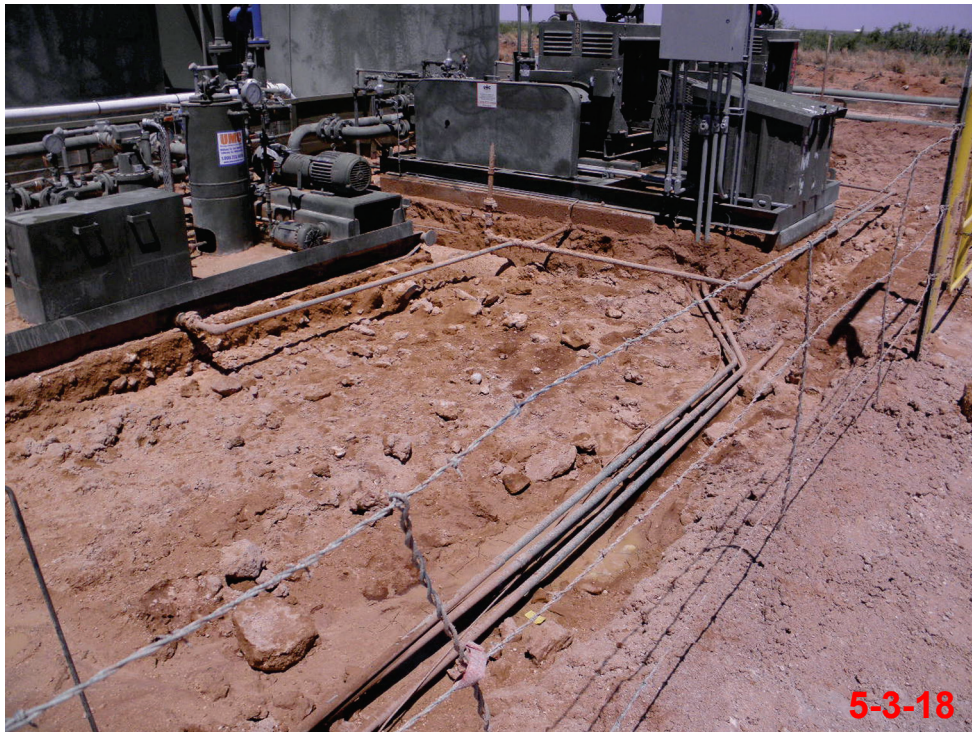
Photo 11 - View of hydrovac activity along southern edge of LACT Unit facing east
