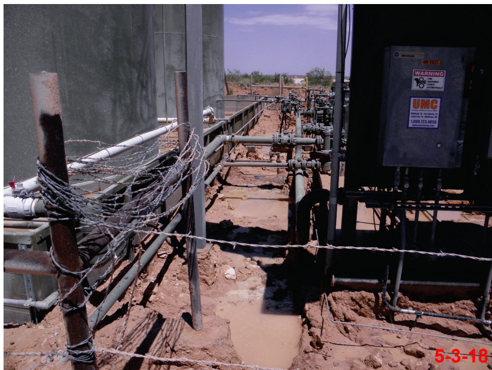
Photo 9 – View of hydrovac activity along northern edge of LACT Unit facing east
