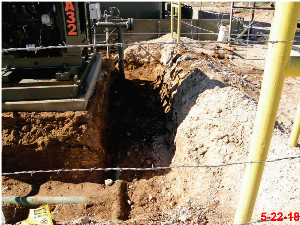
Photo 16 – View of hand digging activity along eastern edge facing north
