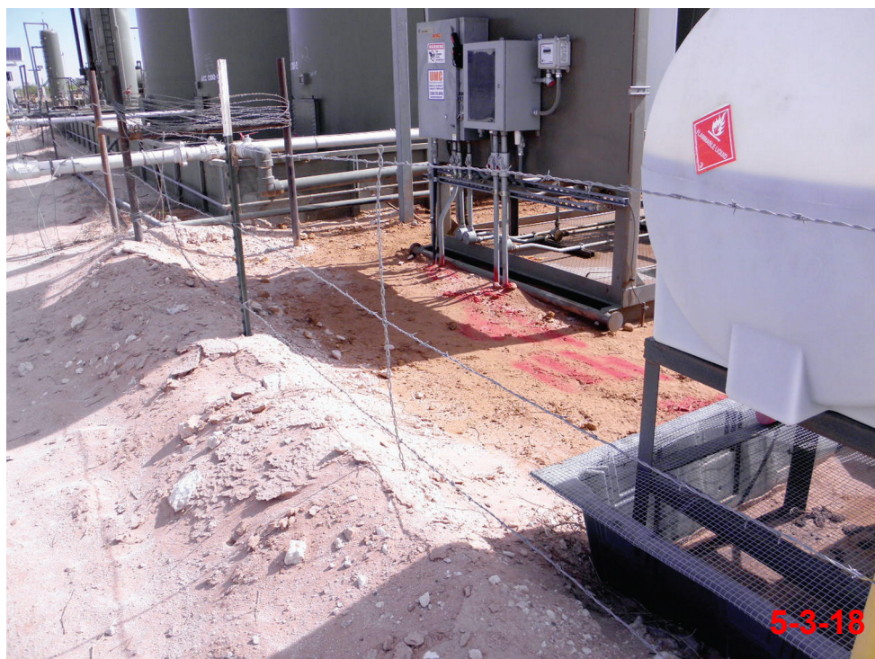
Photo 8 – View of impacted soil along western edge of LACT Unit facing north-northeast
