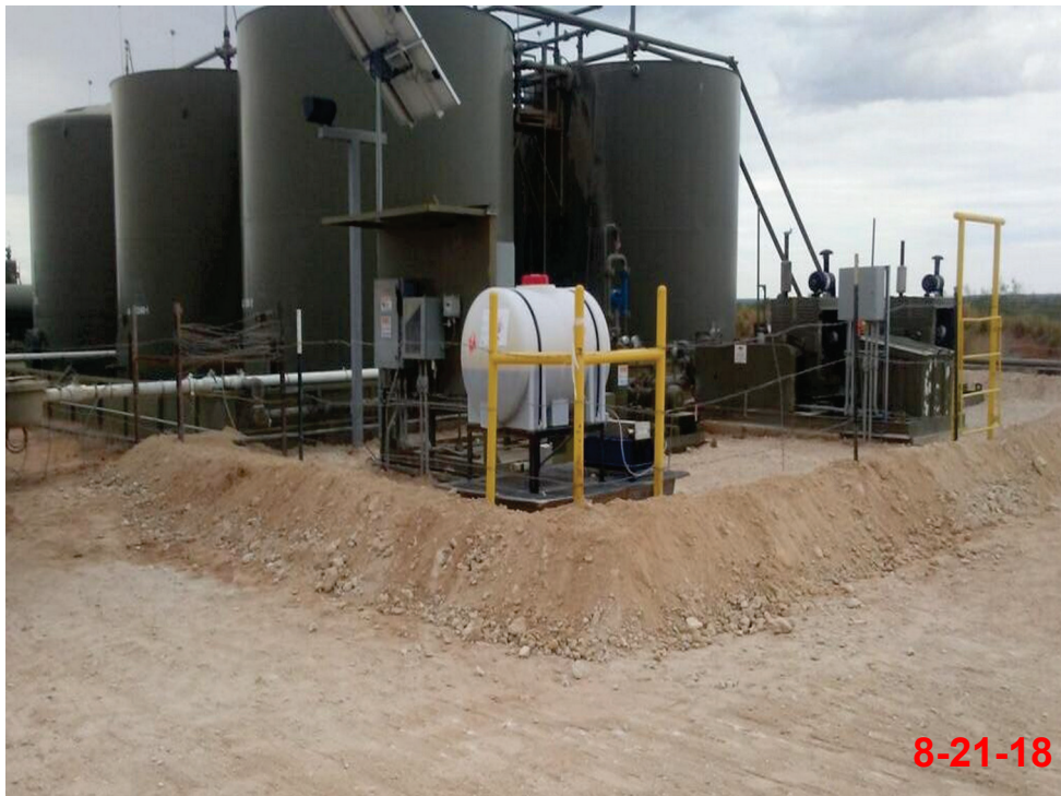
Photo 18 – View of backfilled and restored LACT Unit area
