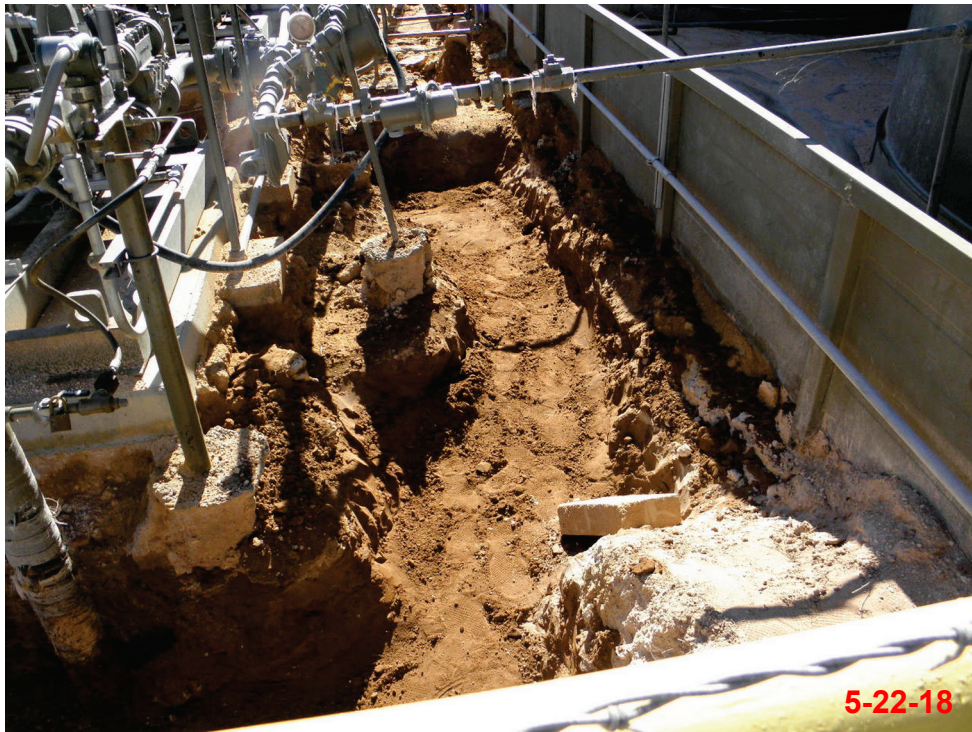
Photo 17 – View of hand digging activity along northern edge facing west
