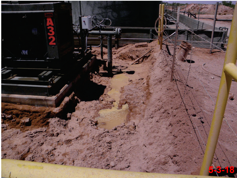
Photo 14 – View of hydrovac activity around eastern edge of LACT Unit facing north
