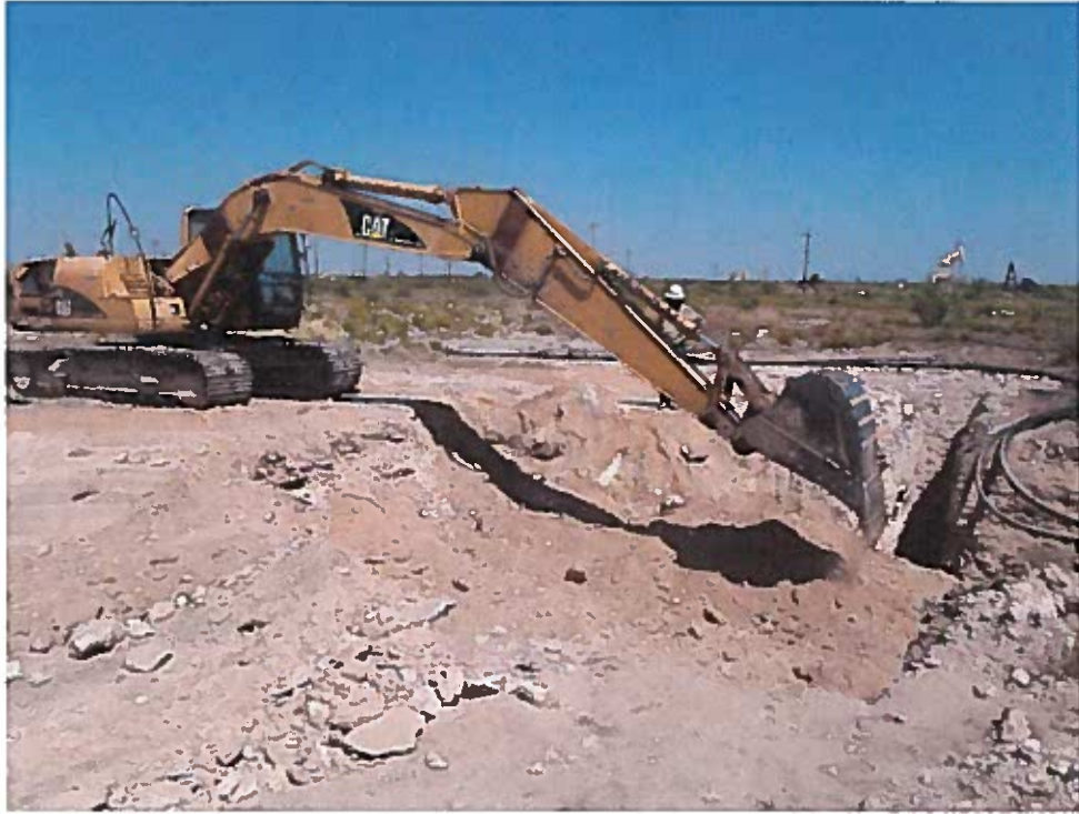
Photo of Backfilling Excavation to 4 feet
