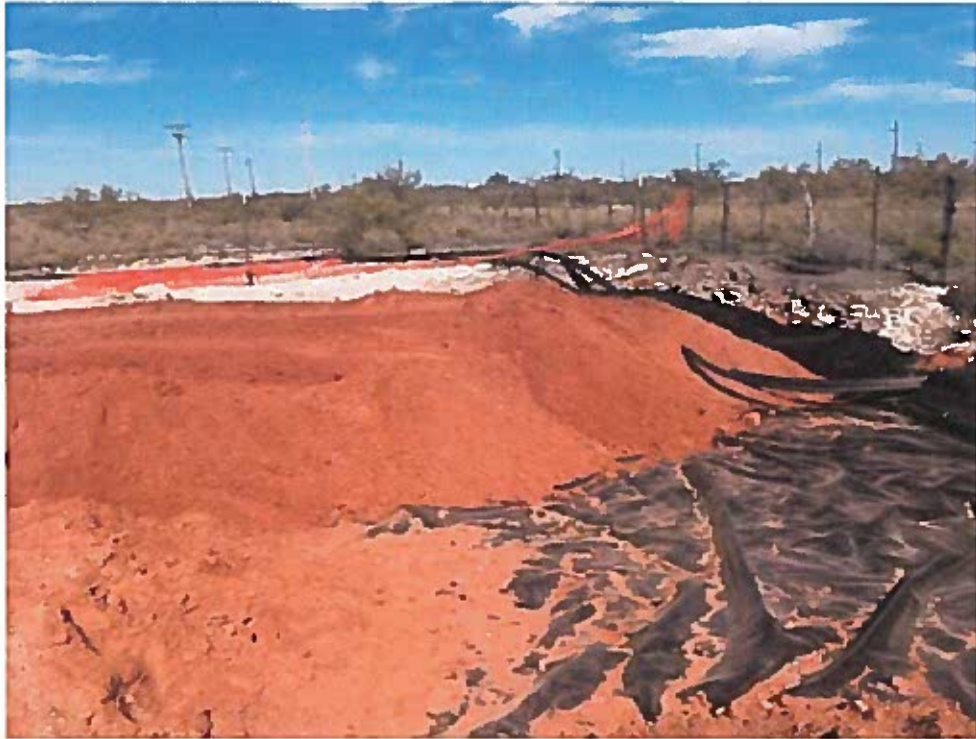
Photo of Backfilling 4 Foot Liner
