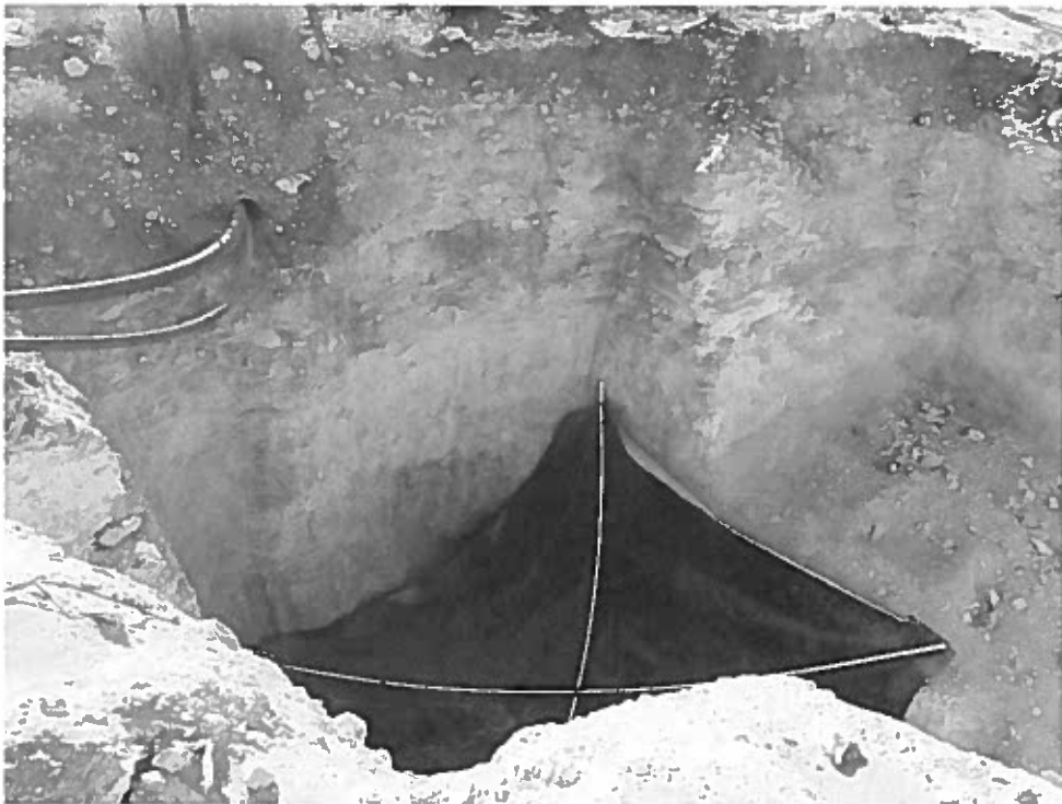
Photo of Liner Installed
