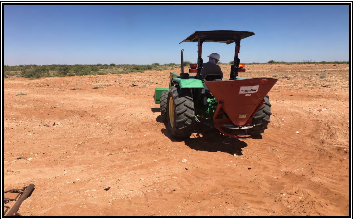
View looking southwest of excavation backfilled to grade, contoured, and reseeding beginning.
