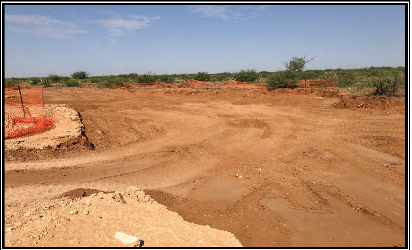
View looking southwest of 20 mil plastic liner covered with clean backfill sand in excavation.
