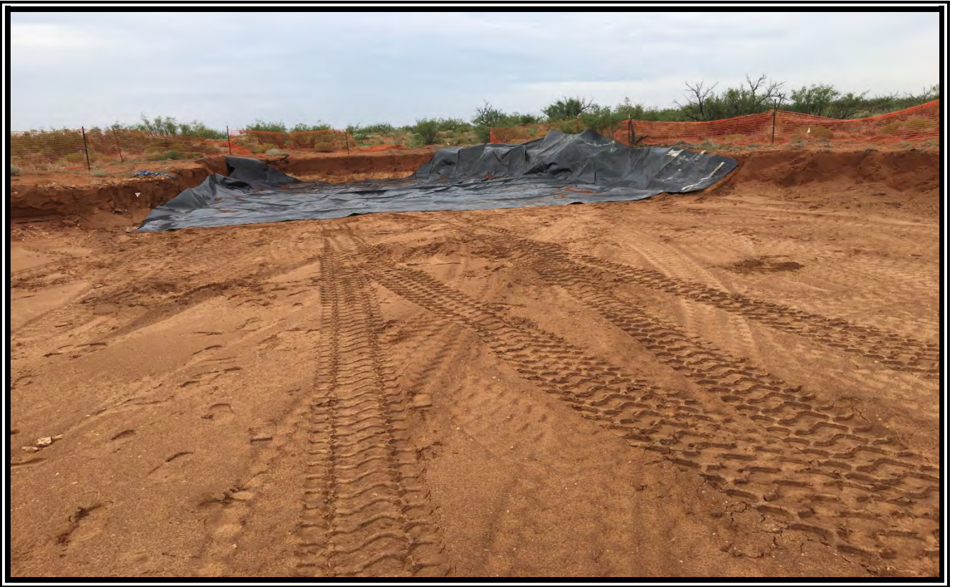
View looking southwest of installing 20 mil plastic liner over emplaced clean backfill sand in excavation.
