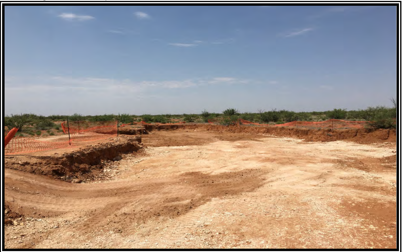
View looking southwest of emplacing clean backfill sand over caliche in bottom of excavation.
