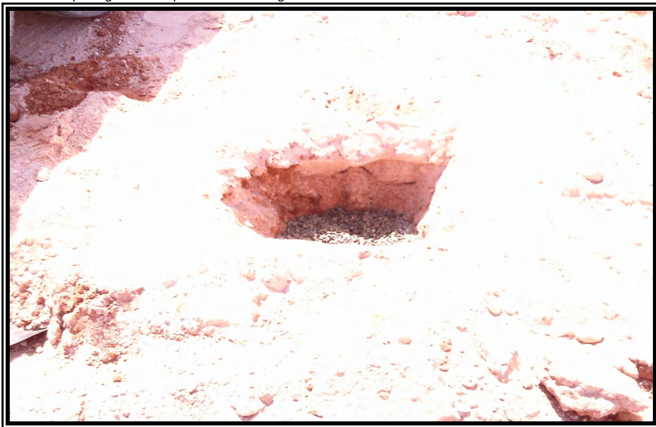
View of soil boring filled with bentonite pellets.
