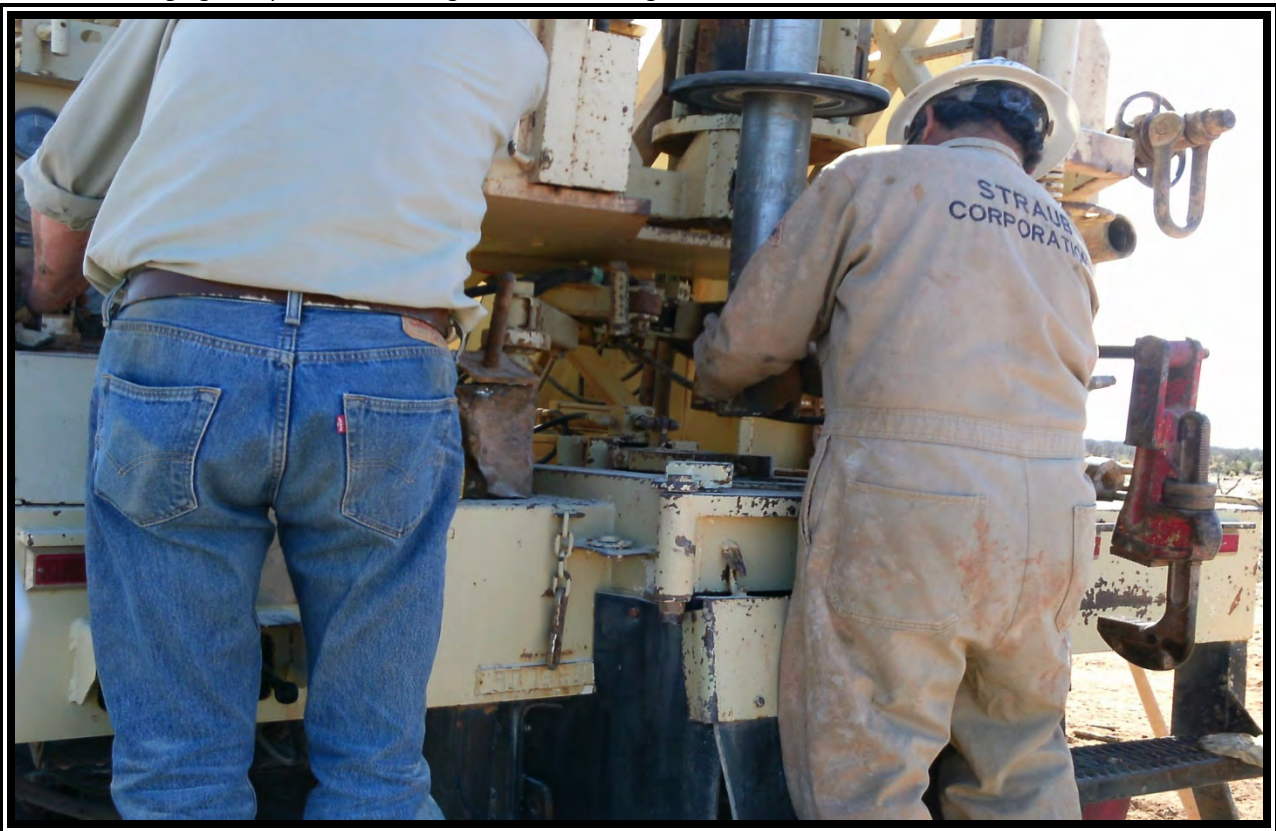
View of plug sampler being attached to drill string.
