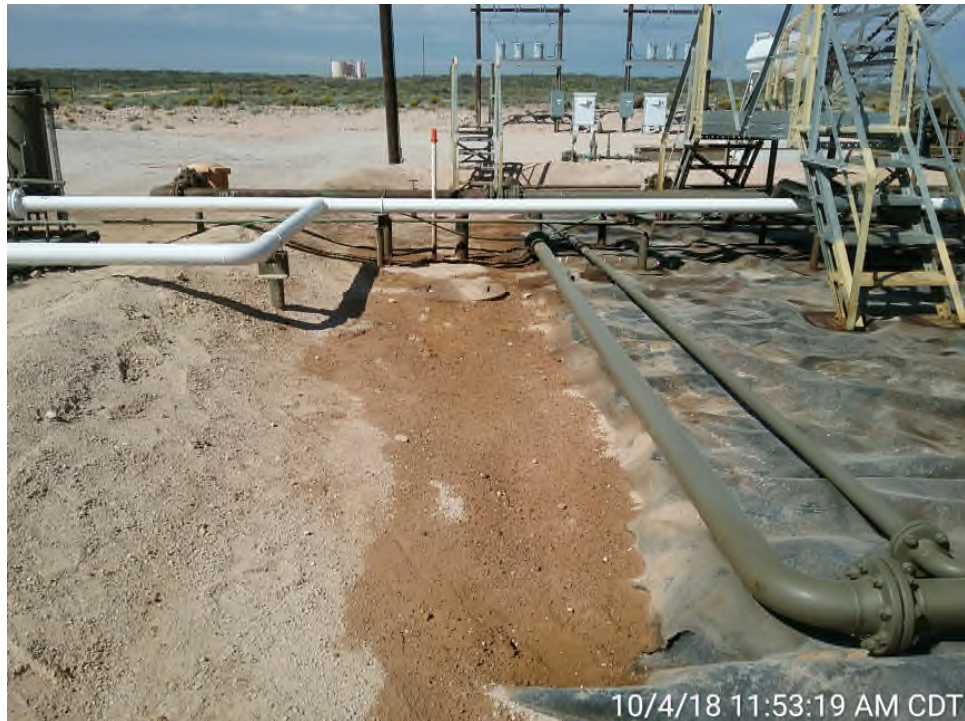
View facing North – Spill area
