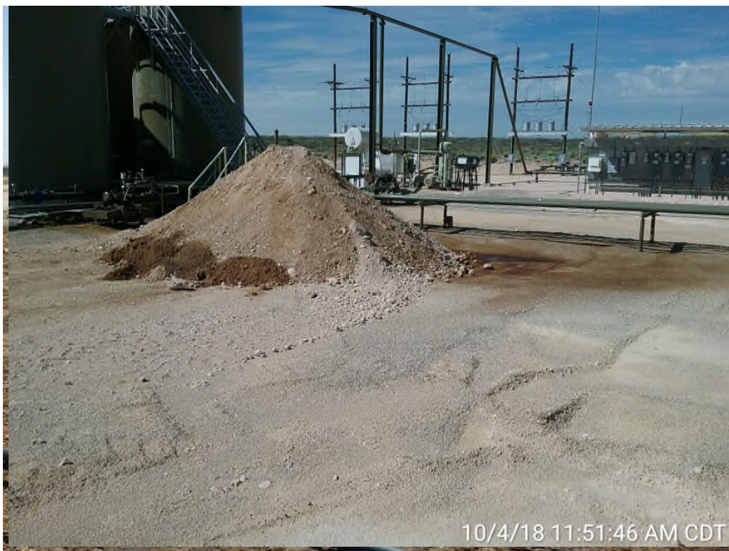
View Southwest – Spill area containing soil removed from emergency excavation
