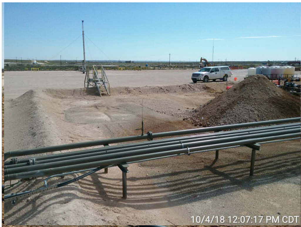
View Southeast – Spill area containing BH-4, BH-5, BH-6, and BH-9
