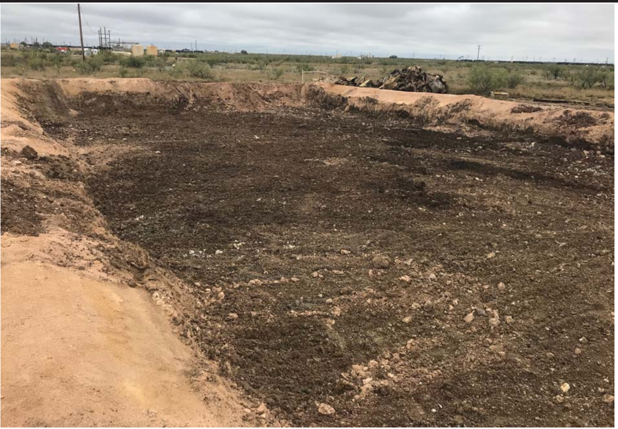
Figure 7 - View of affected area after excavation activities, facing North.
