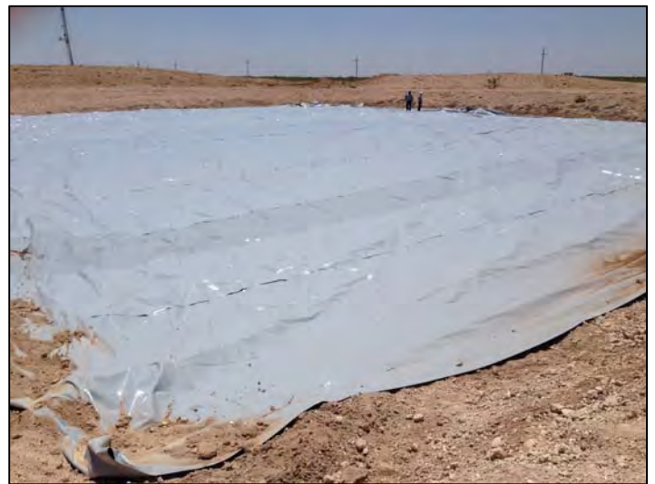
Liner Installation Complete 6-26-2014
