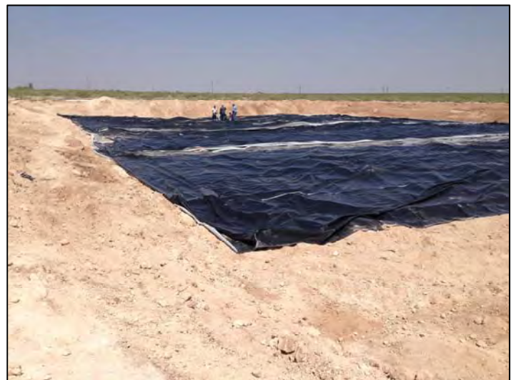
Installing geomembrane cover 7/24/2014
