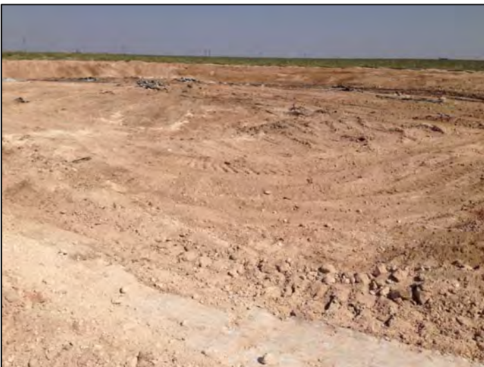
Stabilized cuttings 4 feet below surrounding grade 7/24/2014
