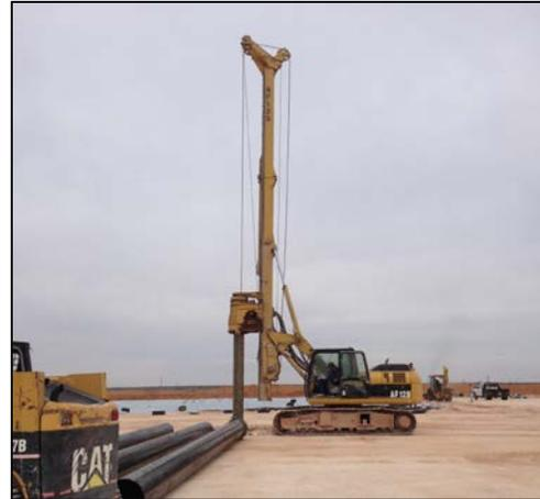
On March 3<sup>rd</sup> and 4<sup>th</sup>, 2014 I witnessed the drilling of the conductor hole for the Bettis 20 State Com 2H well, located in eastern Lea County. Ready Drill LLC of Monahans, Texas performed the work using a track-mounted 30-inch auger drilling rig as shown in the photograph above.
