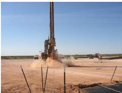
The photograph to the left was taken from the soil recovered at a depth of 50 feet as it is being spun from the auger. This photograph demonstrates the lack of moisture in the cuttings. It is believed that any
