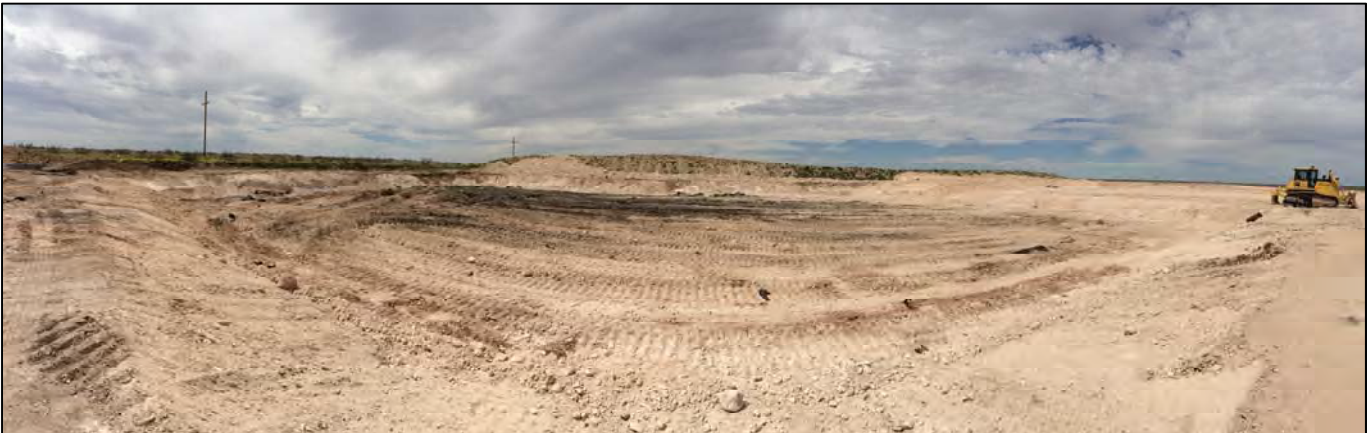
Stabilized cuttings staged for geomembrane cover 4/6/2015
