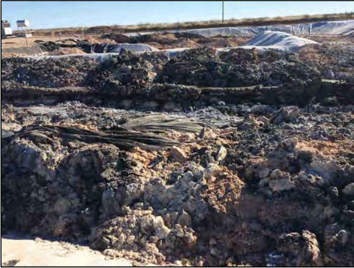
Stabilization mixing of pit contents 1/20/2015
