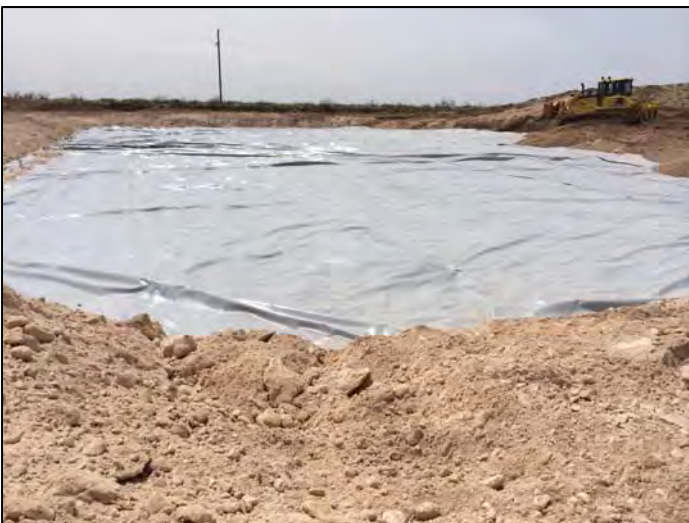
Stabilized cuttings staged for geomembrane cover 4/6/2015
