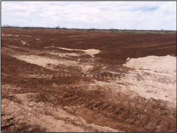
Spreading topsoil over backfilled site 3/25/2015
