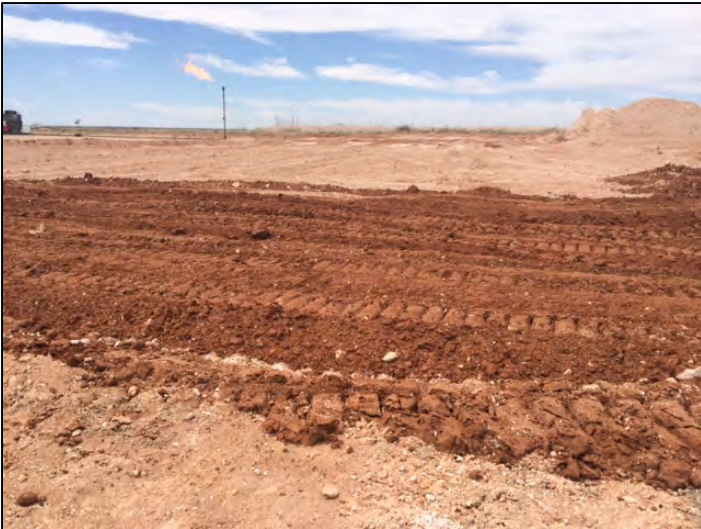
Spreading topsoil on surface 3/25/2015
