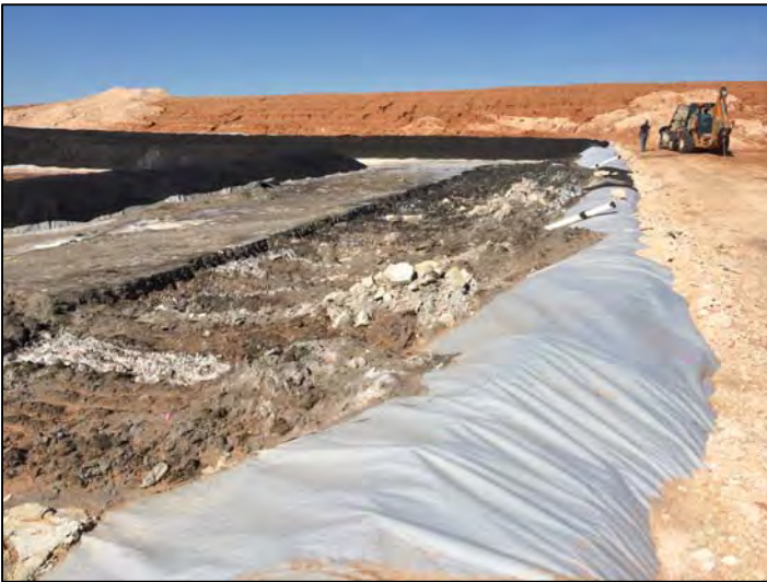
Cutting liner at mud line 2/13/2015
