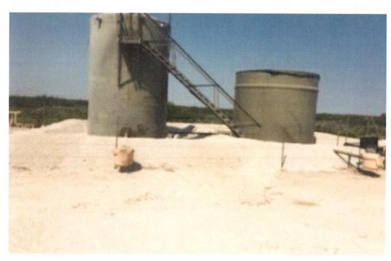
40 mill liner inside herm and covered up with dirt
