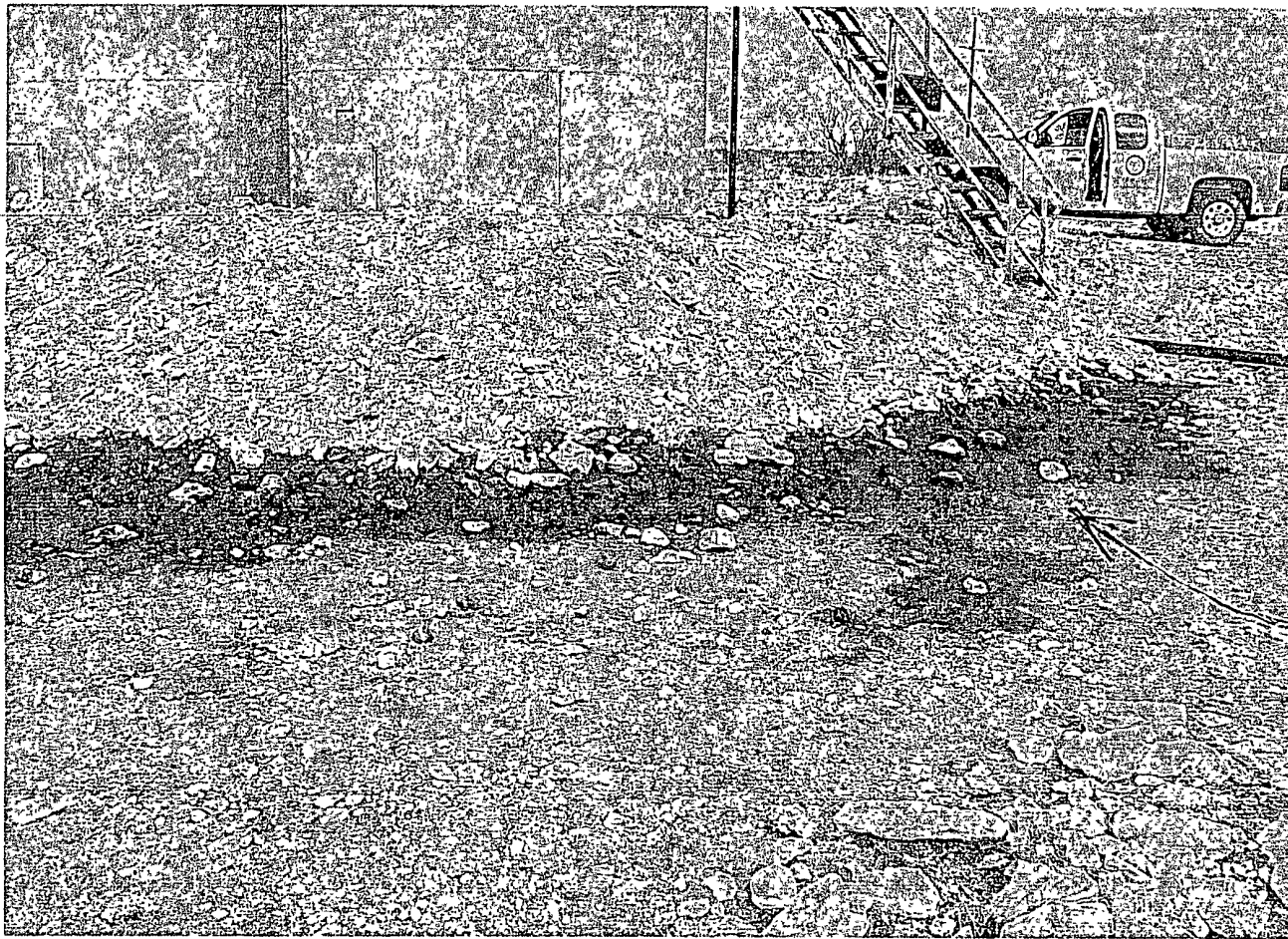
LEAK THROUGH BERM
