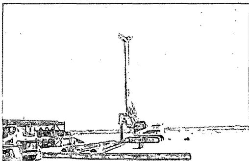
On February 27, 2013 Dale Littlejohn witnessed the drilling of the rat hole at the Mogi 9 #1H site. Ready Drill LLC of Monahans, Texas performed the work using a track-mounted 30-inch auger drilling rig as shown in the adjacent photograph.
