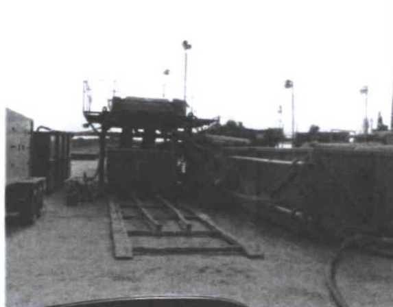
Above: Centrifugal Closed Loop System
