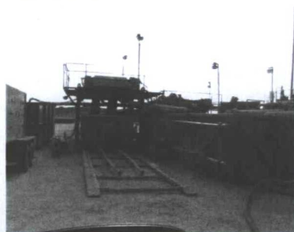
Above: Centrifugal Closed Loop System
