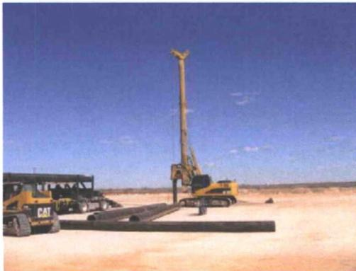
On February 27, 2013 Dale Littlejohn witnessed the drilling of the rat hole at the Mogi 9 #1H site. Ready Drill LLC of Monahans, Texas performed the work using a track-mounted 30-inch auger drilling rig as shown in the adjacent photograph.
