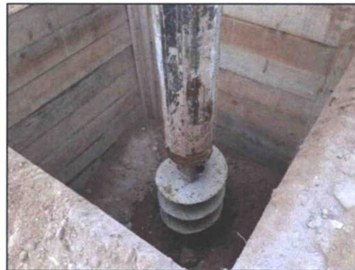
Over the next 6.5 hours the boring was advanced to a total depth of 120 feet by removing approximately 1.5 feet of material per trip into the hole. I inspected the cuttings from each trip for moisture to indicate a groundwater formation, but all samples were dry. If any appreciable moisture would have been indicated, the operation would have been suspended to allow the water to accumulate and then measured.
