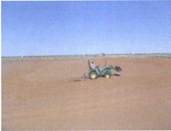
Initial discing of site
