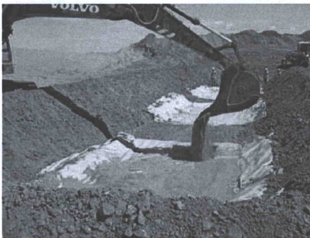
Figure B-2: Installation of leak detection liner panels and permeable material over panels
