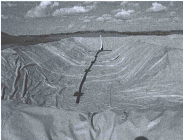
Figure B-6: Lined pit with dewatering system installed
