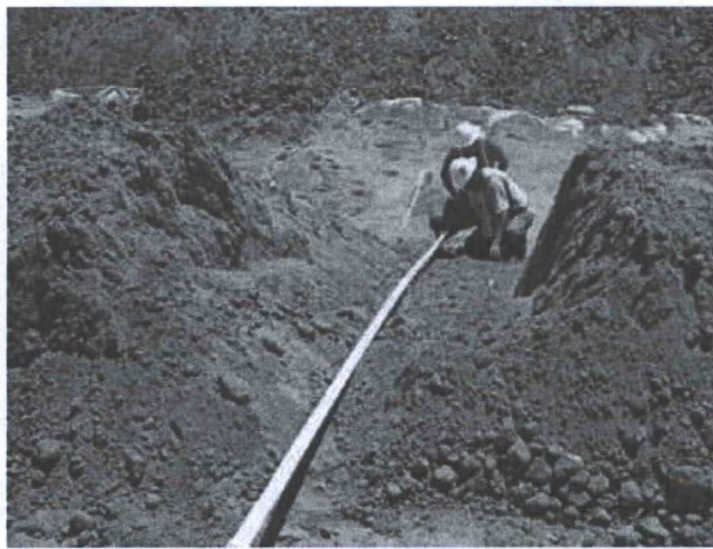
Figure B-4: Placing conduit from moisture sensor to ground surface
