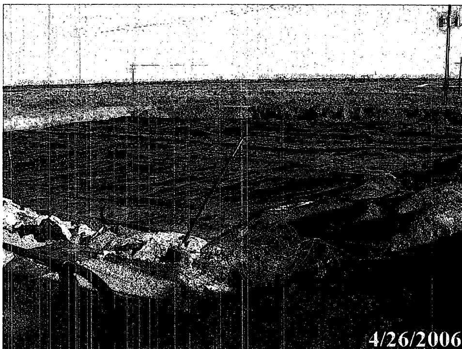
Photograph #3 – Liner covering stiffened pit contents.
