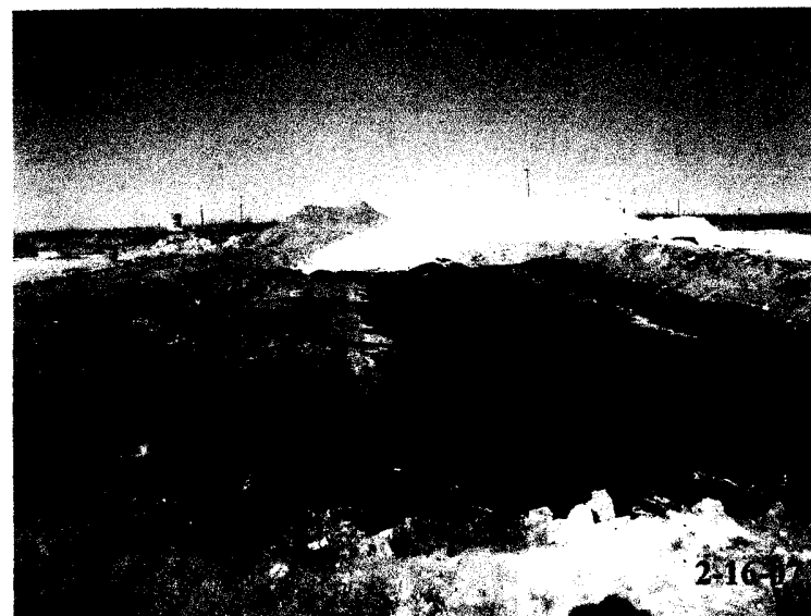
After 20 mil impervious lining of drilling pit for risk based closure.
