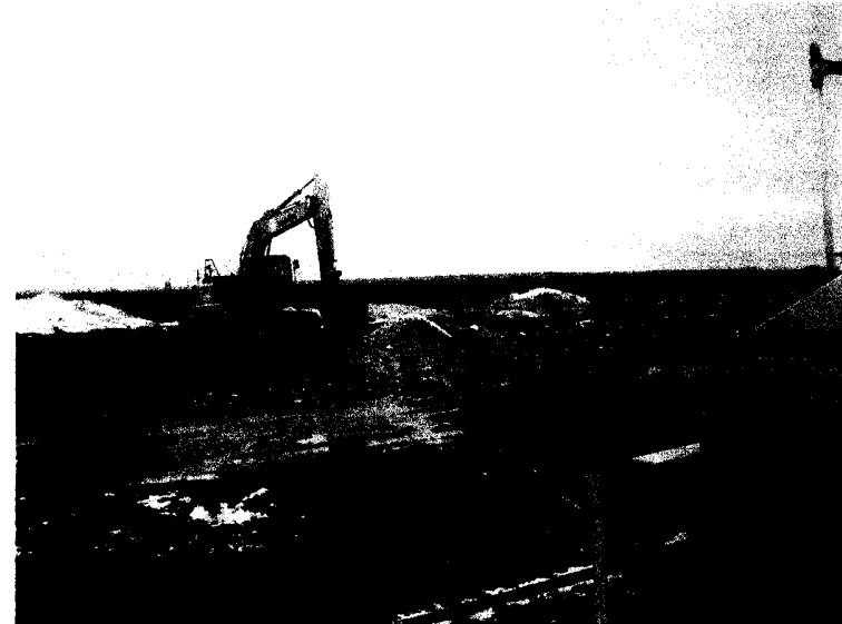
Solidification of contamination for risk based closure.
