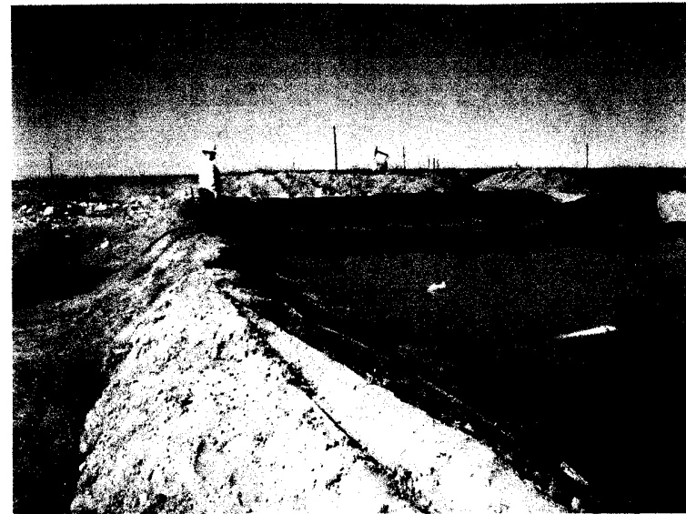
Removal of excess water from drilling pit.
