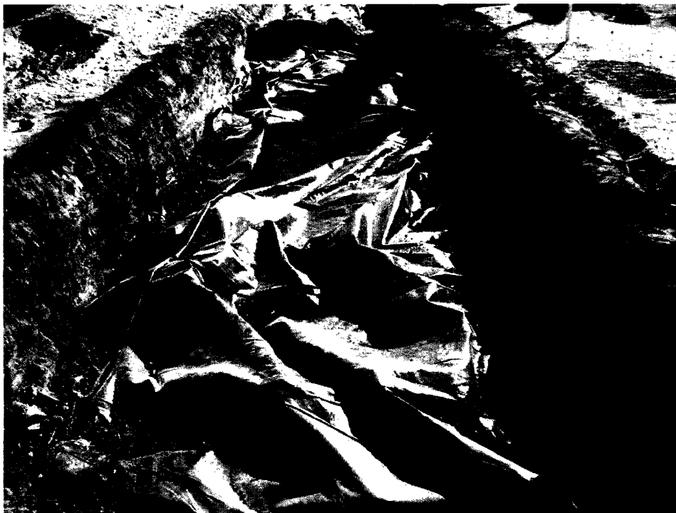
Photograph #5 – Liner covering stiffened pit contents.
