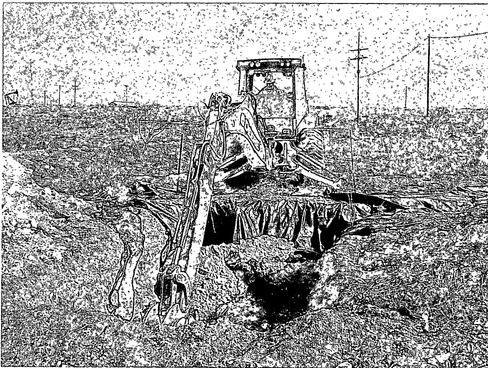
Excavation of mud and liner.
