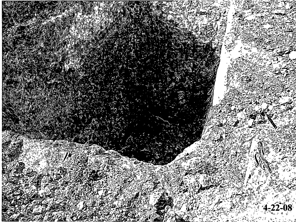
Site after excavation of mud and contaminated soil @18' bgs.
