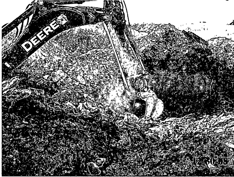
Excavation of impacted soil below workover pit.
