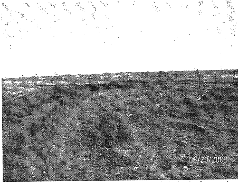
Photograph No. 5 – Stockpiled impacted material within barb wire fence enclosure
