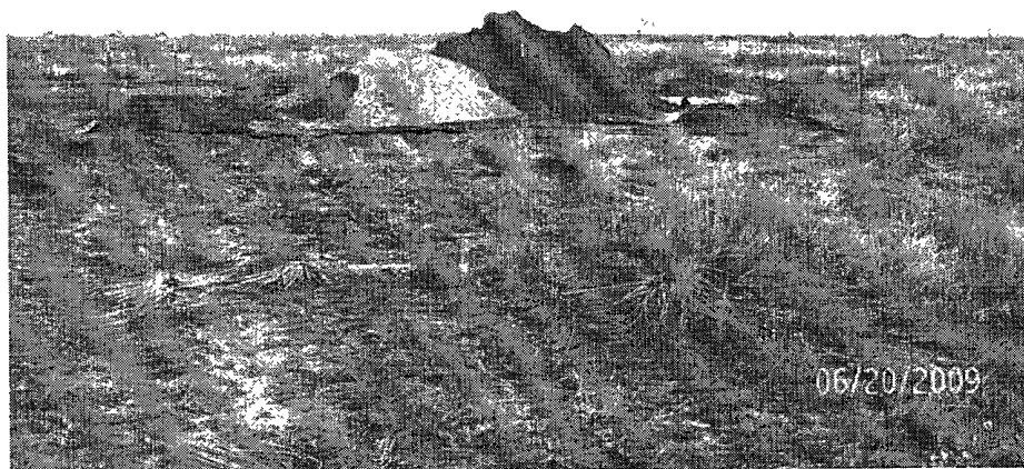
Photograph No. 3 – Impacted material stockpiled on plastic liners
